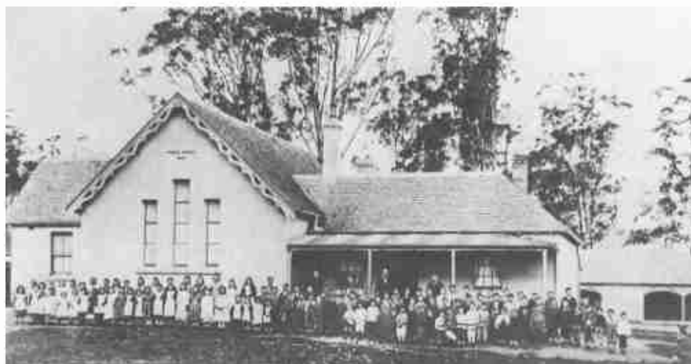
LEICHHARDT PUBLIC SCHOOL: the 1849 building (left wing)
