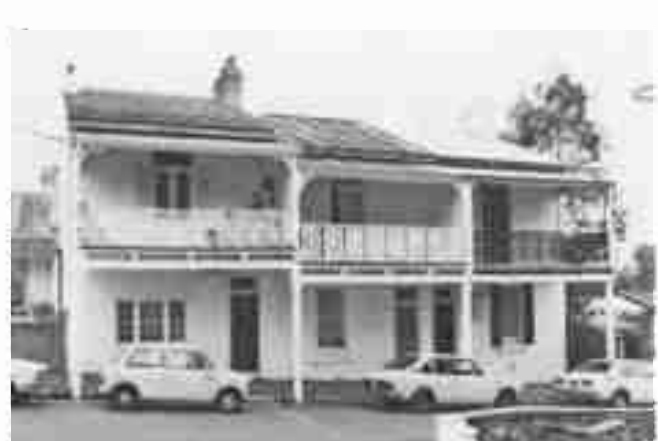
15-17 East Street, Balmain
