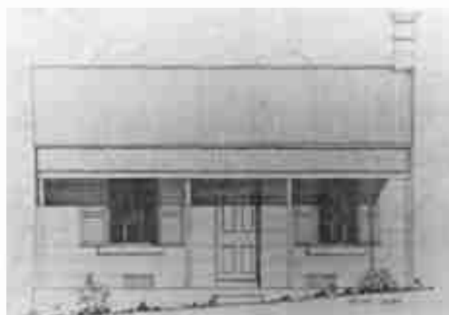
8 99-118A (2211011); 1 Carrington Street John Cavill leased the land from A.W. Reynolds in 1908
