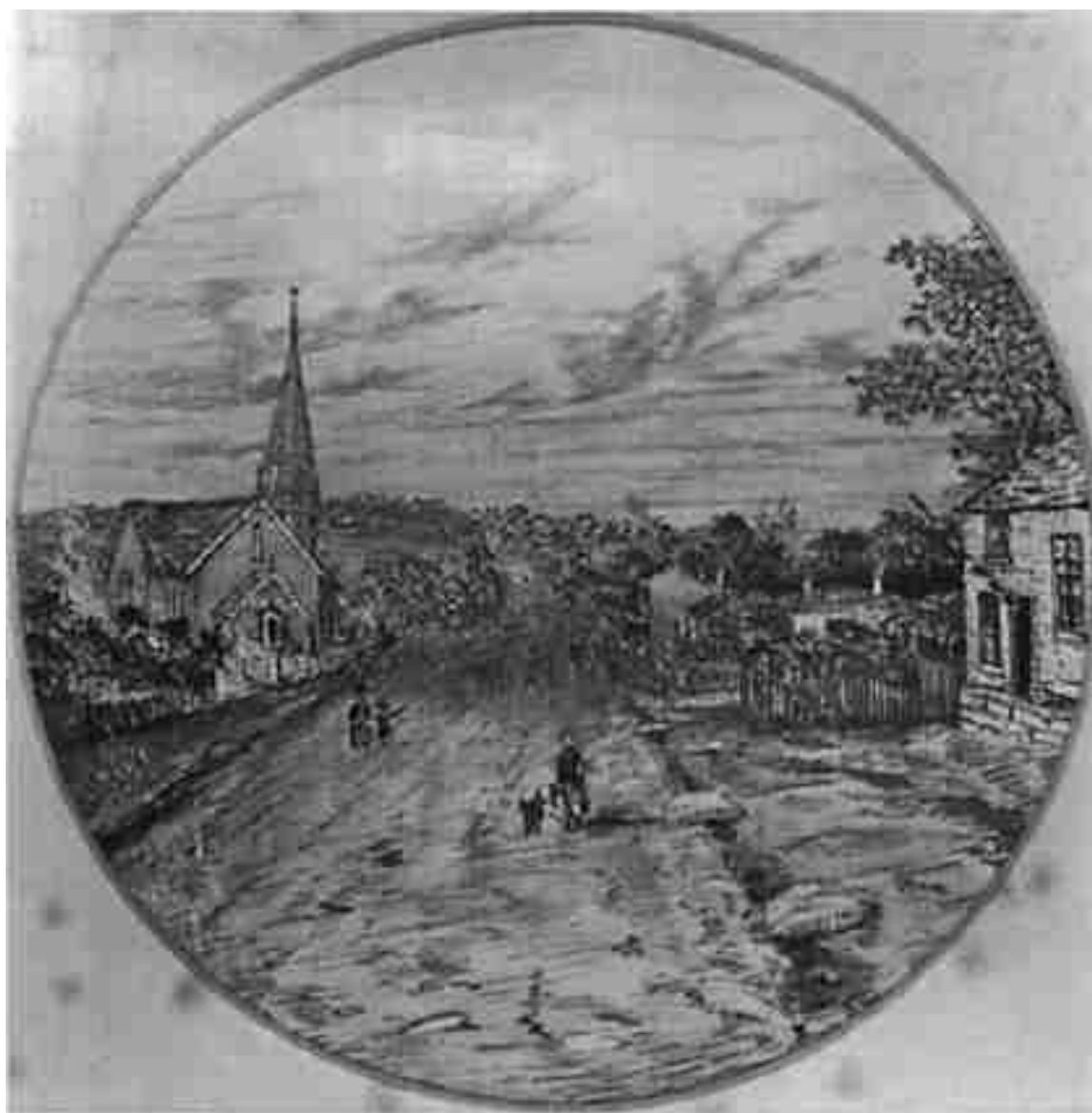
Second Balmain Presbyterian Church, 1857 James McDonald, Architect
