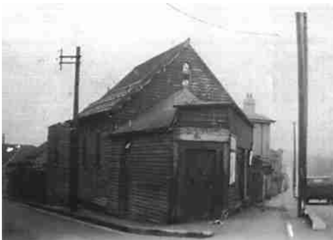
The Dilapidated Condition of the Church/shop Before its Demolition
