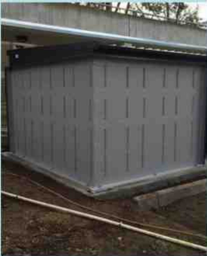
Waterproofing for a green wall (Source: Bravada, 2019)
