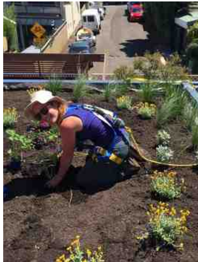
Extensive green roof, Rozelle (source: 202020 Vision, 2018)
