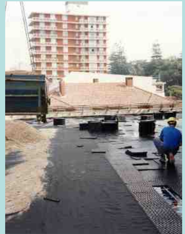
Green roof in construction, Manly (Source: Atlantis, 2008)
