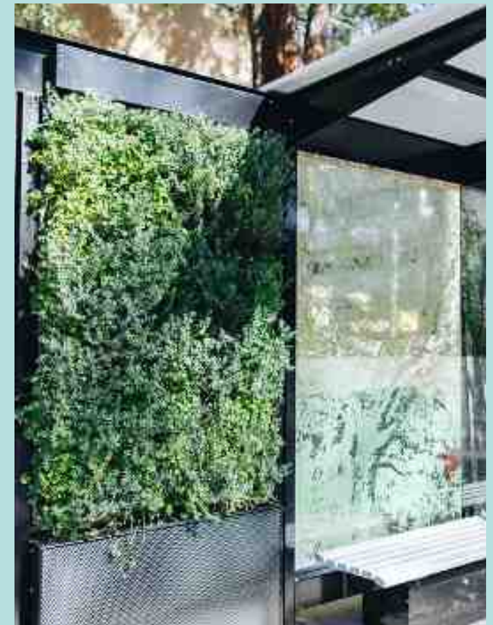
Green wall, Macquarie Park bus shelter (source: Junglefy, 2018a)
