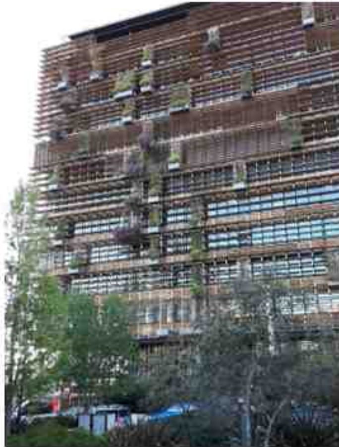
Green facade using cable system with planter boxes, Nishi Building, Canberra
