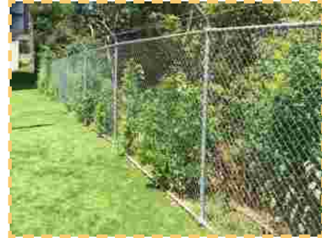
Chainwire mesh fencing
