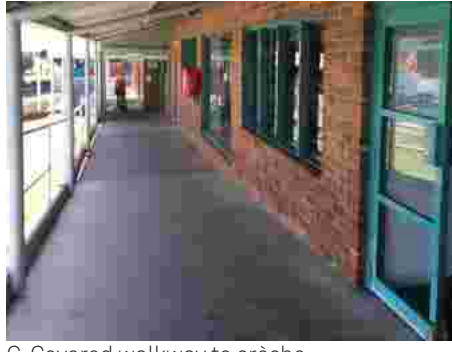
C. Covered walkway to crèche
