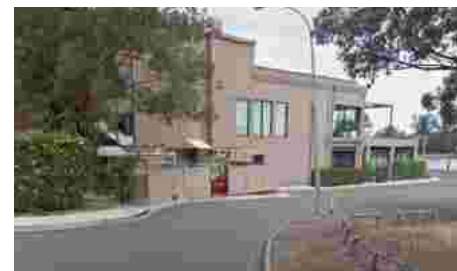
B. Disconnected footpaths between Le Montage and the project site.
