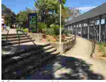
A. Entrance ramp and stair access
