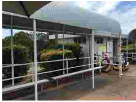
Awning to pool surrounds
