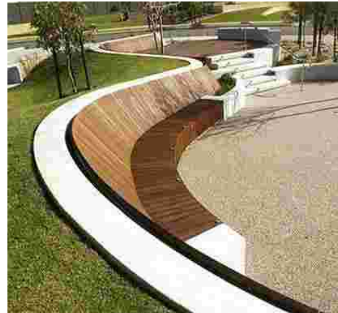
Combination of concrete and timber seating
