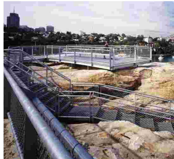
Ballast Point Park - chain mesh balustrades
