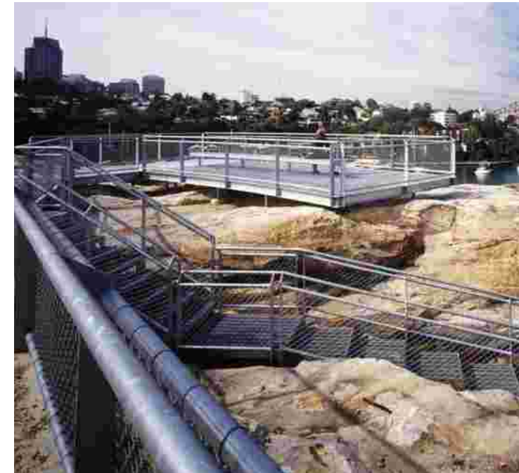
Ballast Point Park - chain mesh balustrades
