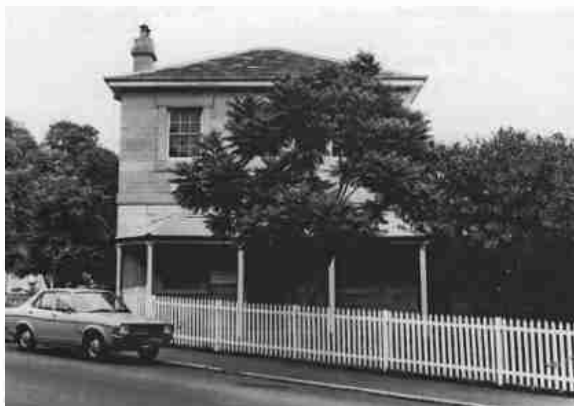
4.10: The Balmain Watch House, 179 Darling Street, 1854, 1881
