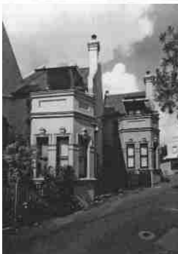
3.27–3.28: 5–7 Colgate Avenue, 1898 Known locally as the Concertina Terraces, the small houses, built by Samuel Weirick, maximise the site. (B Cresson)
