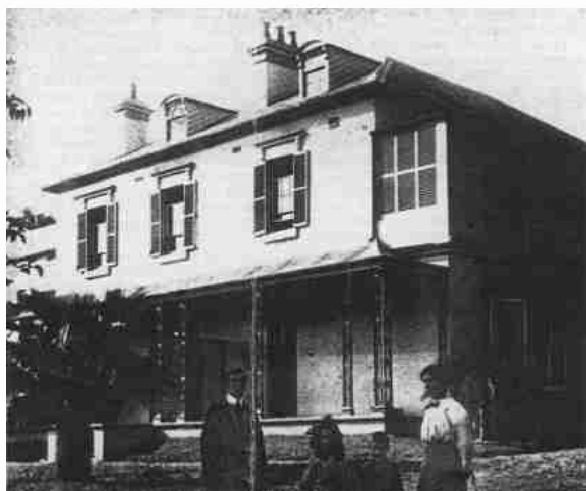
Glenwood at 57 Hereford Street in c1913
