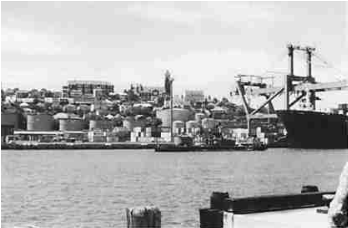
Containerisation Operating, Oil Tanks Remaining 1979
