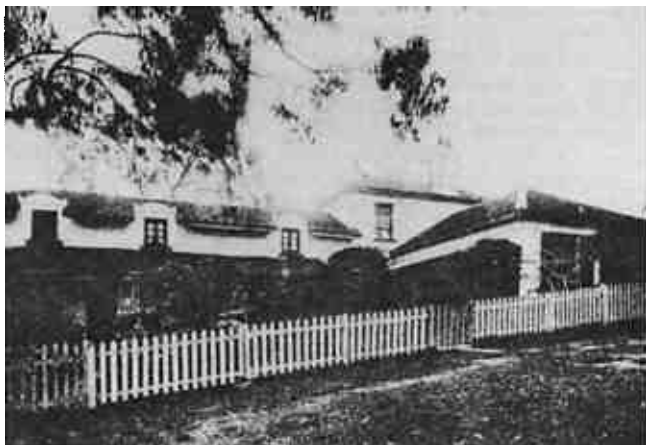
LOOKE'S COTTAGE IN 1902. (Australian Town & Country Journal, 10 December 1902) Built of stone with timber shingled roof, the cottage (now 15 Lookes Avenue) had unusual upper-storey windows with parapets.
