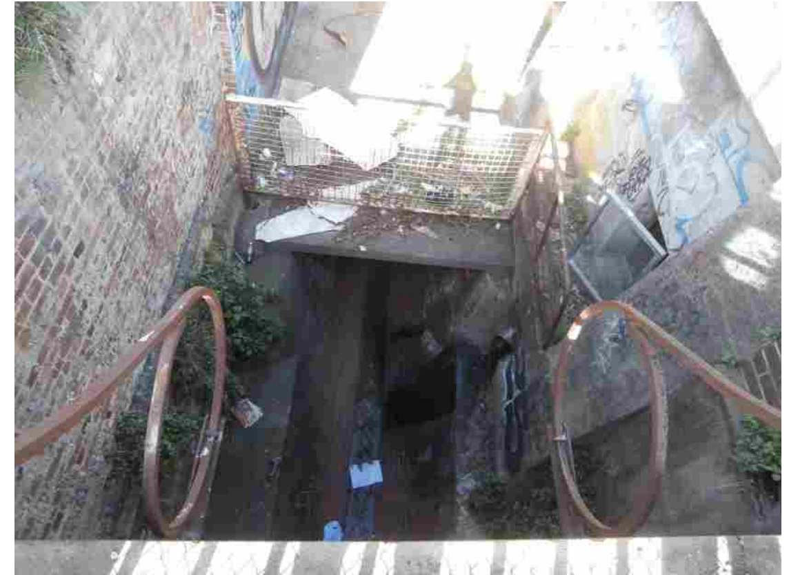
Above: Johnstons Creek upstream of Parramatta Road
