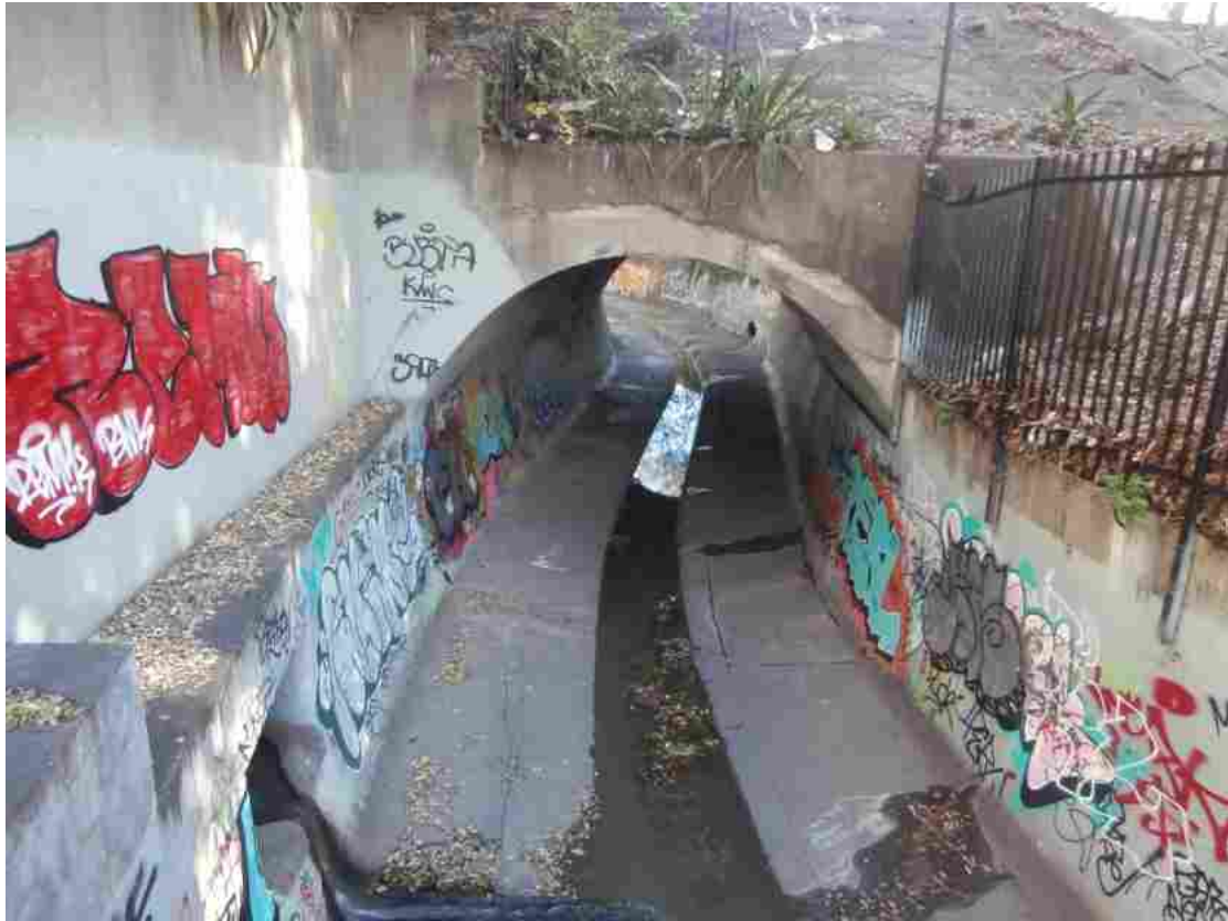
Above: Johnstons Creek downstream of Booth Street
