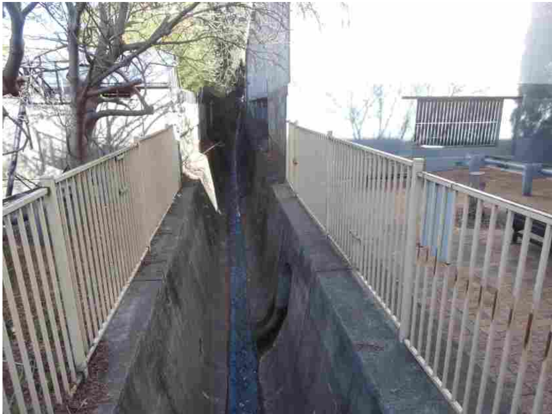
Above: Johnstons Creek upstream of the Cruikshank Street Pedestrian Bridge
