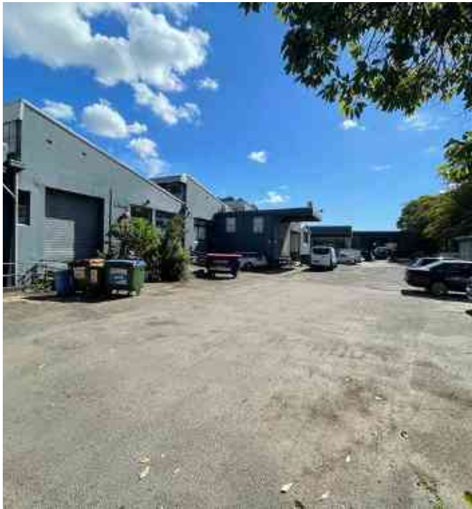
6. Eastern Facade and forecourt
