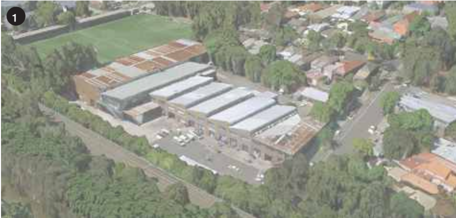
Existing Site Buildings Image - Source: MetroMap 2016
