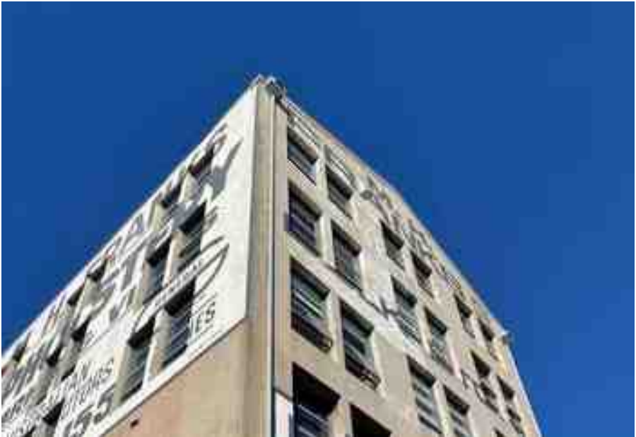
industrial-residential building on Parramatta Road
