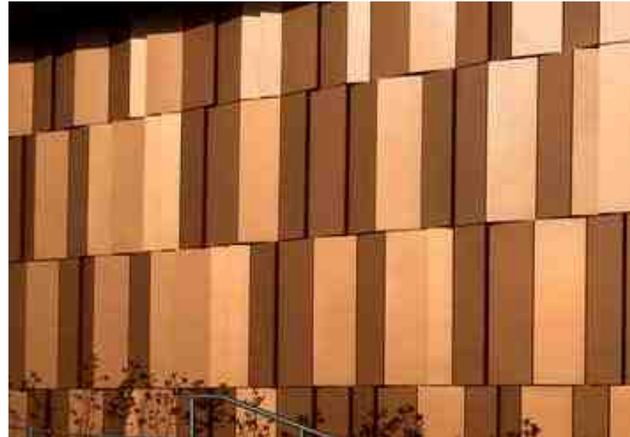
2 copper finish to sun-shading fins
