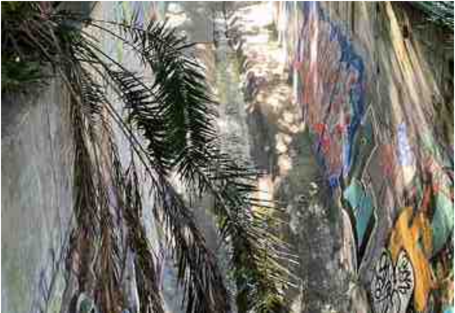
concrete gully along Johnston's Creek
