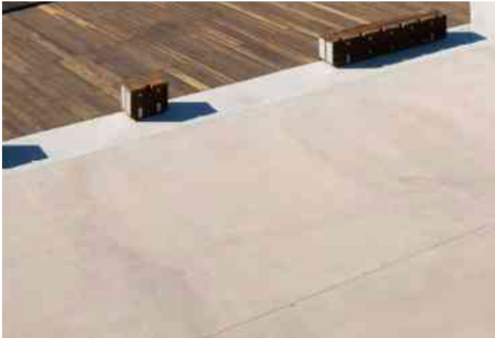
Insitu concrete paving
