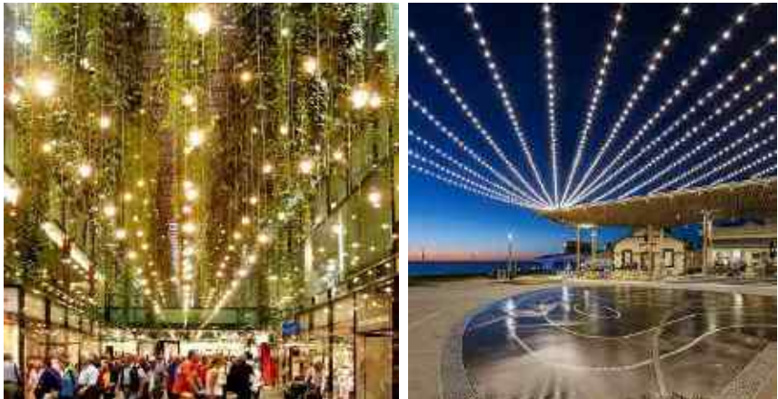
Catenary lighting elements
