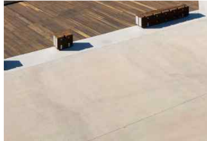
Insitu concrete paving
