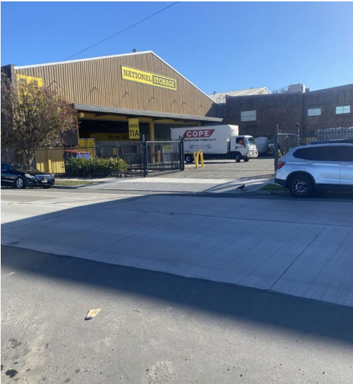
Picture 3 View of the 11A Edinburgh Road site entrance at Edinburgh Road
