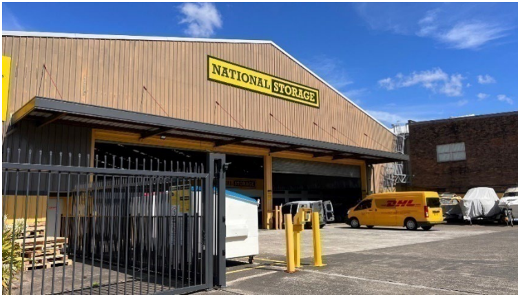
1. National Storage from Edinburgh Road
