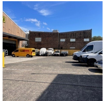
2. Parking & loading area
