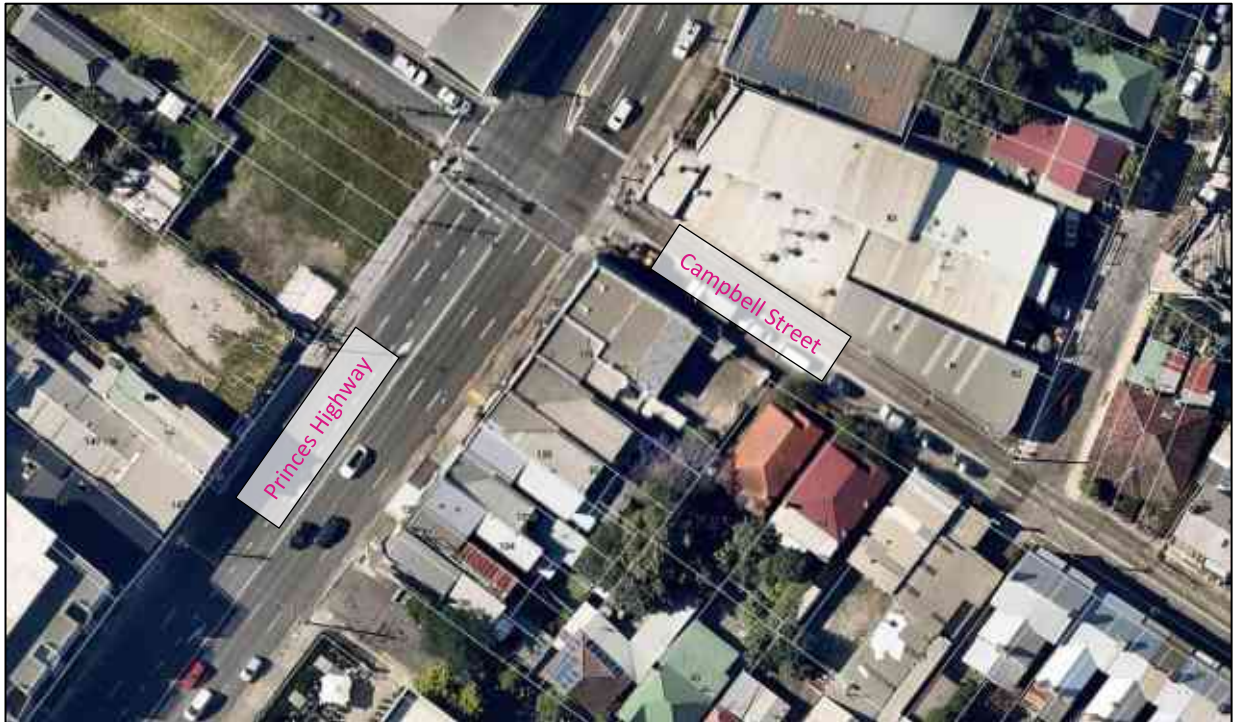
Figure 4 - Princes Highway / Campbell Street before upgrades (31 October 2016)
