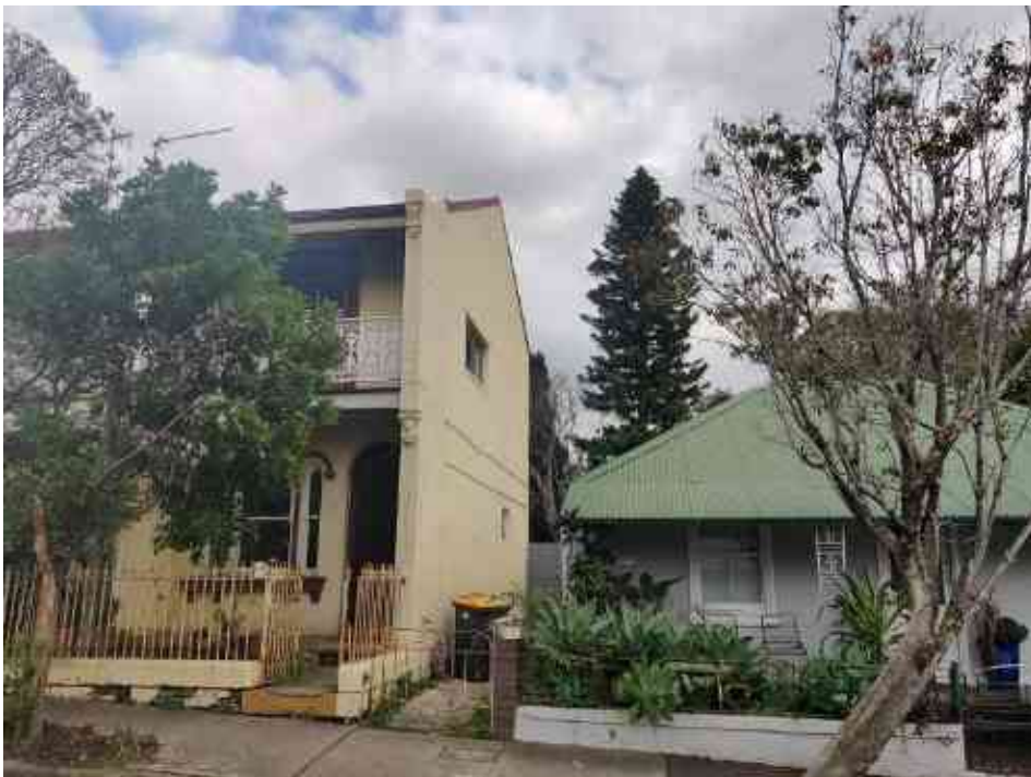
View from Crown Street – site on the left and adjoining house (73 Crown St) on the right side
