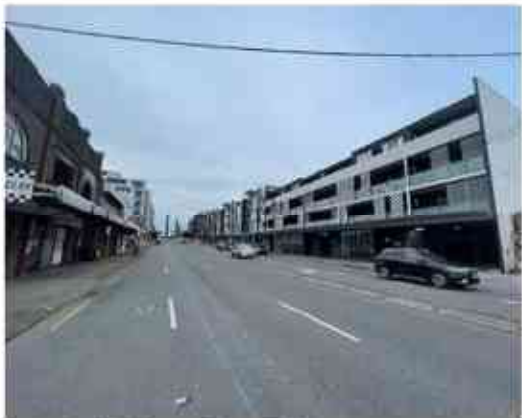
Examples of built form on Princes Highway
