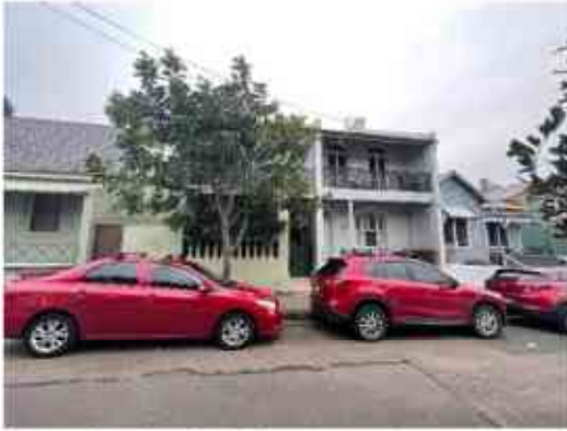
Terraces viewed from Crown St
