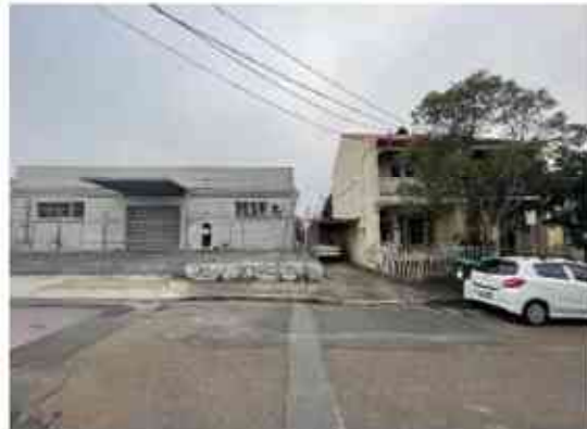
View from Crown Street of 116 Princes Highway (left) and 75 Crown Street (right)
