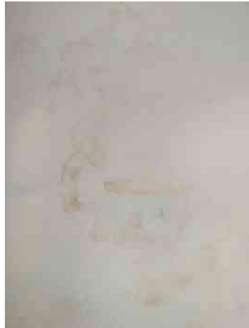
Figure 4-16: Damp damage to plaster at 77 Crown Street. Source: Curio 2023
