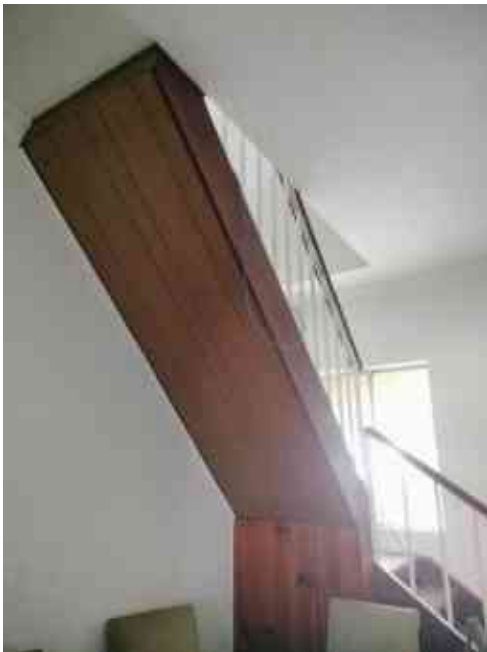
Figure 4-9: Stairwell in 77 Crown Street. Source: Curio 2023
