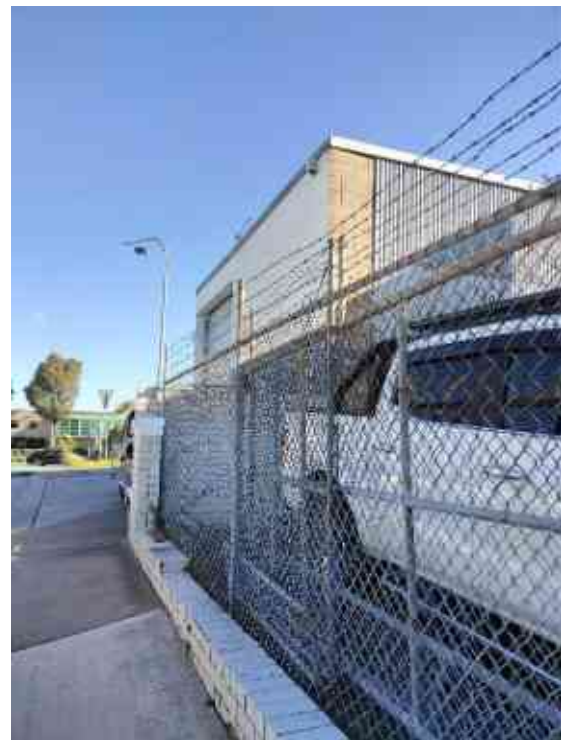
Figure 4-46: Crown Street frontage, facing south. Source: Curio 2023
