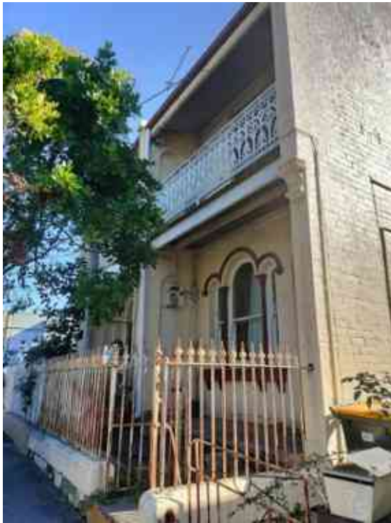
Figure 4-25: 75 Crown Street façade, facing southwest. Source: Curio 2023
