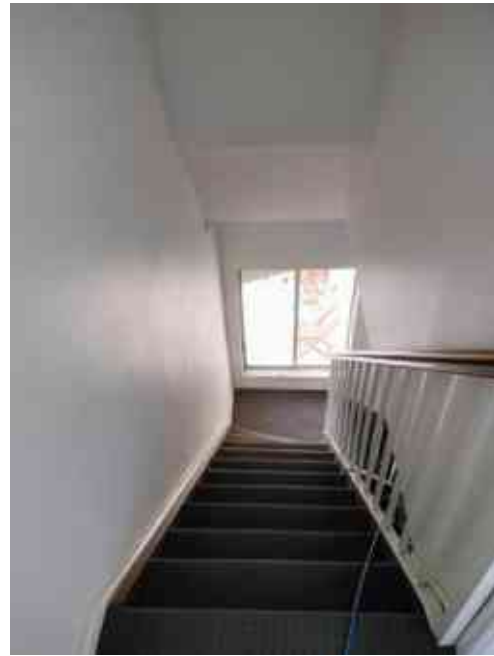
Figure 4-12: Stairwell with modern balustrade. Source: Curio 2023
