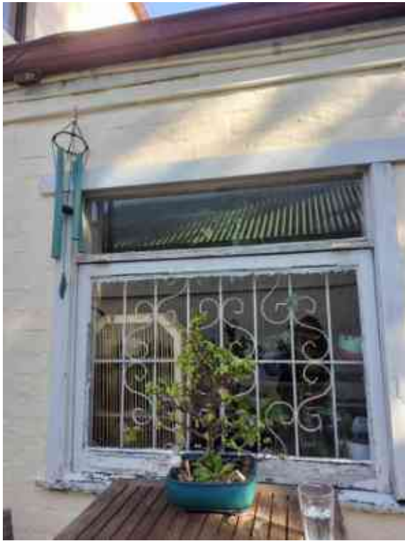
Figure 4-41: Back window of annex. Source: Curio 2023
