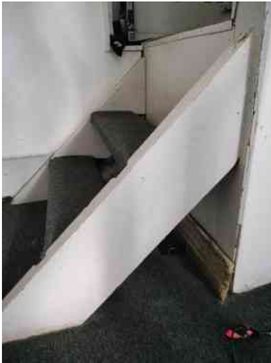
Figure 4-37: Added flight to bottom of stairwell. This area is damp to the touch with visible mould. Source: Curio 2023
