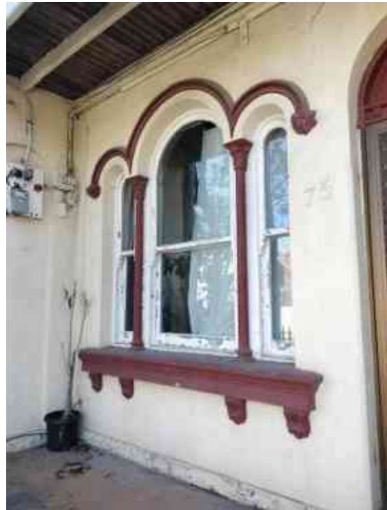
Figure 4-26: 75 Crown Street façade, facing southwest. Source: Curio 2023
