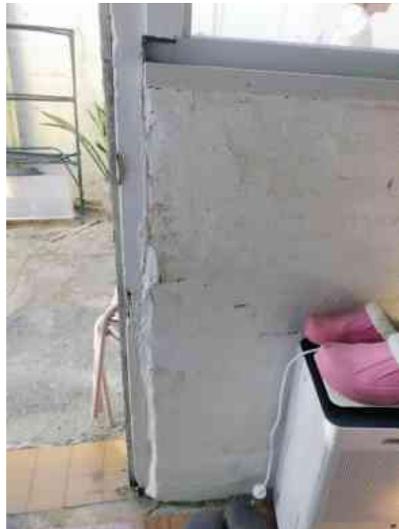
Figure 4-40: Rear door of annex with access into rear yard. Bricks are cracked and inconsistent. Source: Curio 2023
