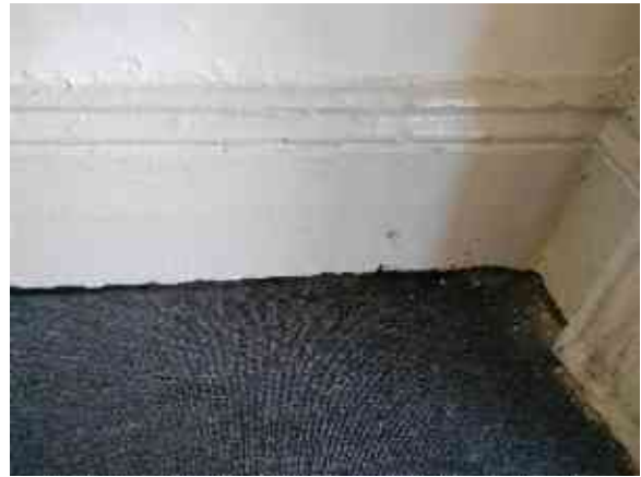
Figure 4-34: Damp damage and wet carpet near front door of 75 Crown Street. Source: Curio 2023
