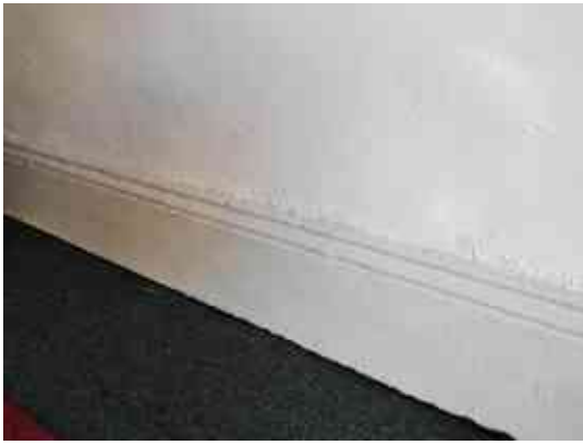
Figure 4-15: Skirting and damp damage to plaster on ground floor of 77 Crown Street. Source: Curio 2023
