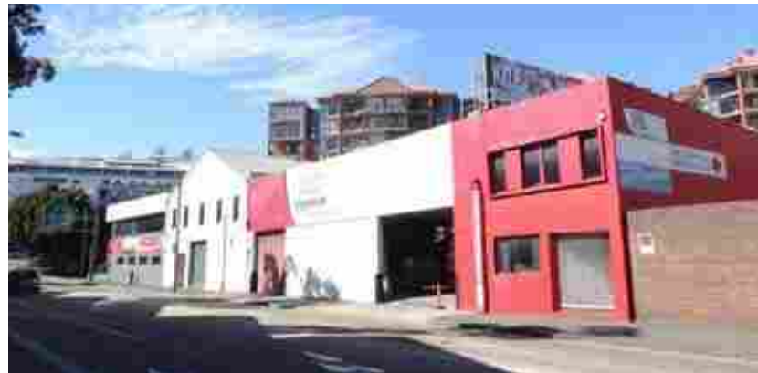
The industrial site before construction of the approved scheme.
