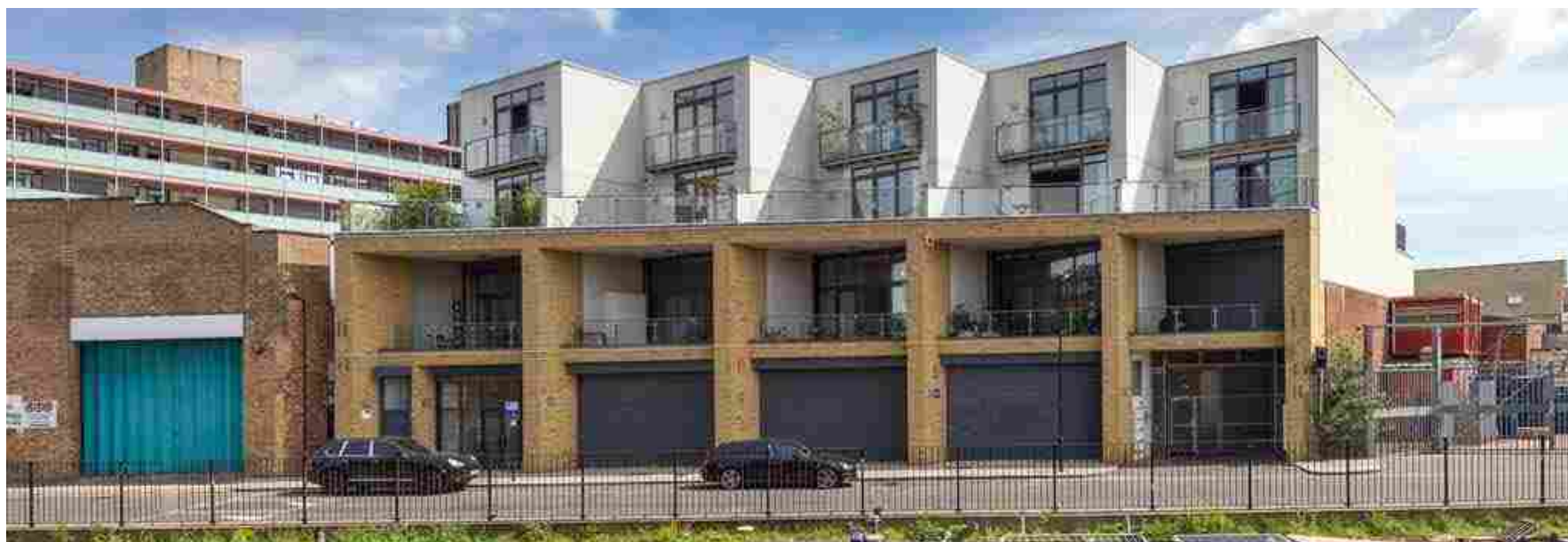
The completed site today showing the entrances to the commercial/industrial ground floor units. The residential entrances are to the rear of the site.
