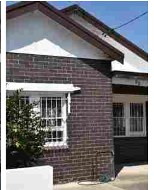
A variety of single storey architectural styles.
