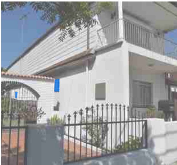
South-eastern wall of 14 Myrtle Street - no habitable windows
