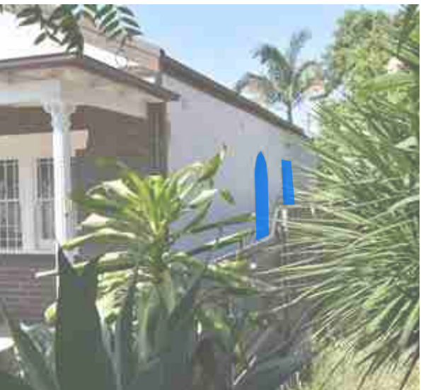
North-western wall of 20 Myrtle Street - no habitable windows
