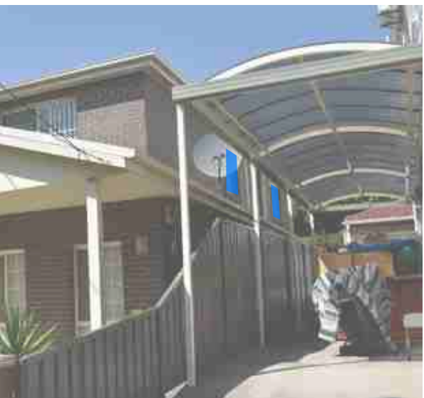
North-western wall of 12 Myrtle Street - no habitable windows
