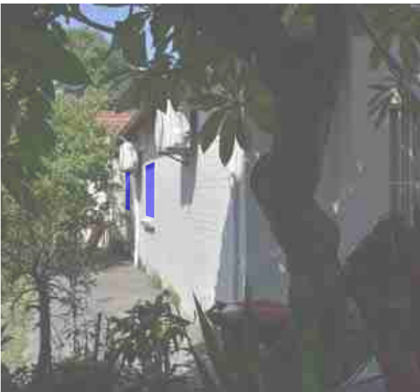
North-western wall of 18 Myrtle Street - no habitable windows
