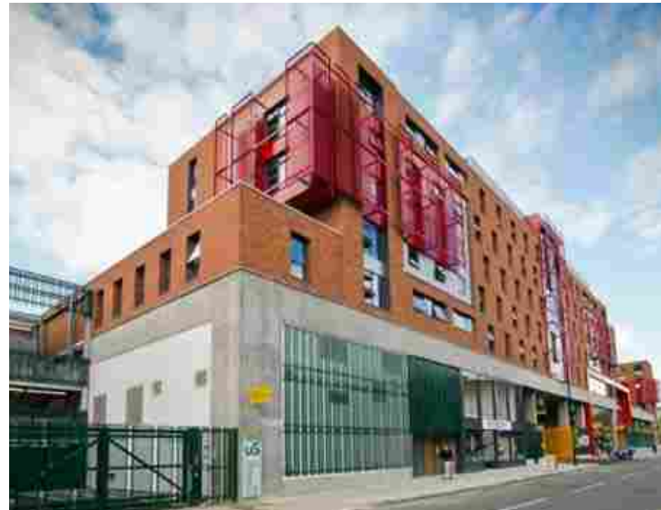
The completed site today.
