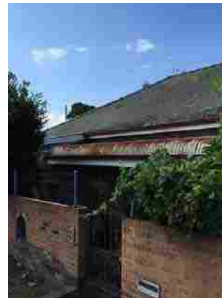
2. Heritage listed stone house 'Loch Lomond' at 1 Myrtle Street adjacent to site. Built in 1860.
