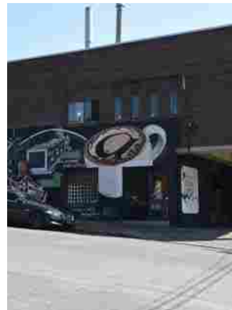
Warehouse buildings with large footprints.
