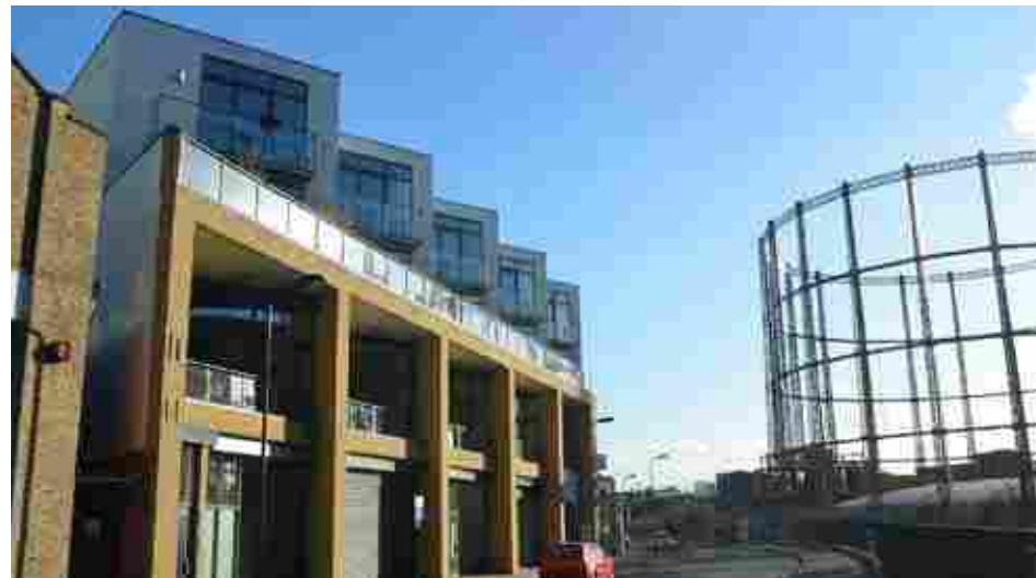
Photograph of completed site today showing the setback from road.
