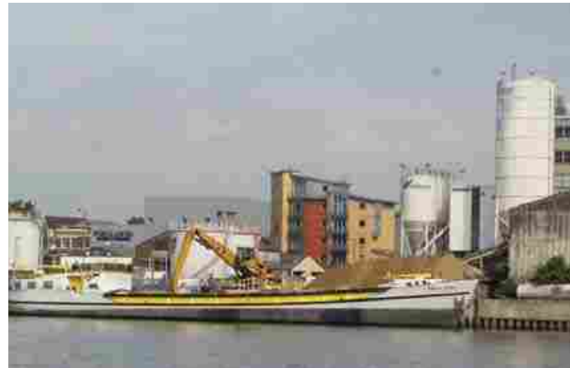
The industrial site before construction of the approved scheme.
