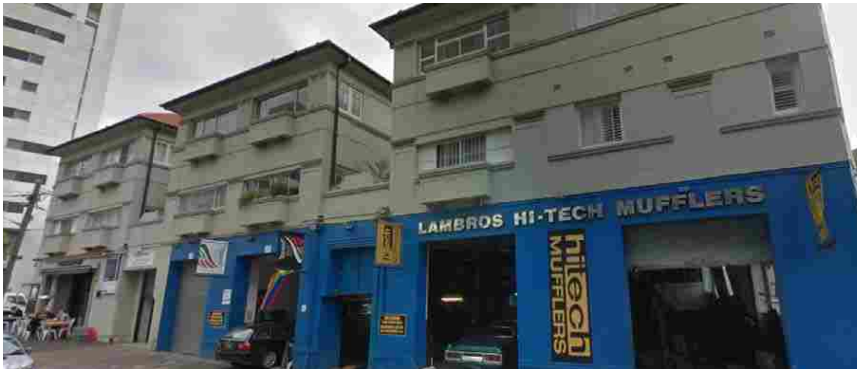
Photograph of the site from street level on Short Street.
