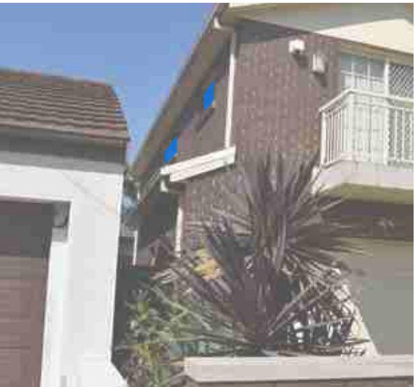
South-eastern wall of 18 Myrtle Street - no habitable windows
