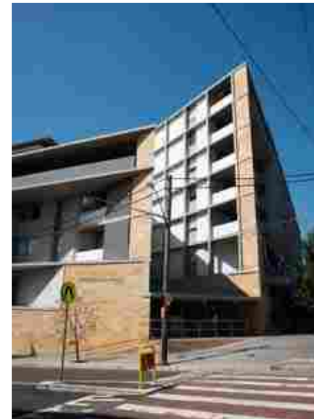
Contemporary residential development
