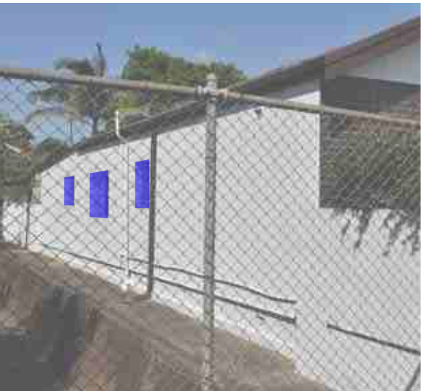
South-eastern wall of 20 Myrtle Street - no habitable windows
