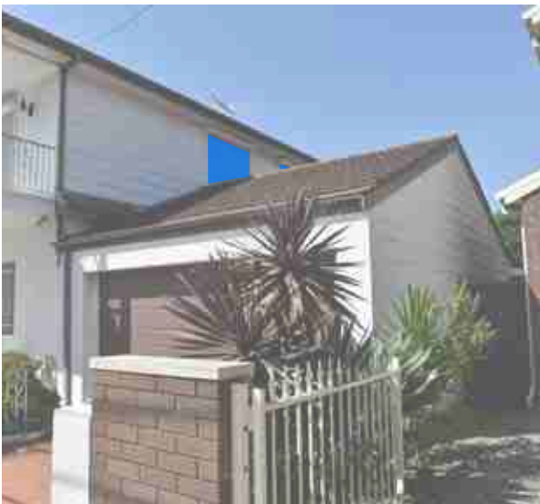
North-western wall of 14 Myrtle Street - no habitable windows
