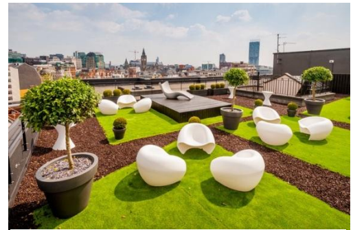
Figure 13: roof gardens help to cool the space and reduce the urban heat island effect.
