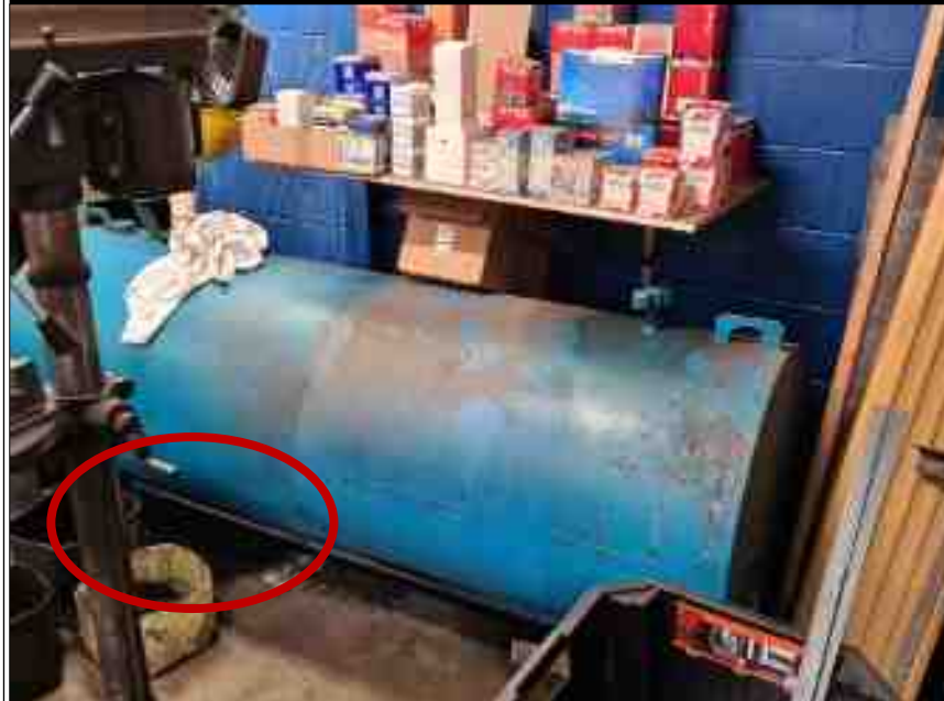
PHOTOGRAPH 4: AST WITH STAINING
