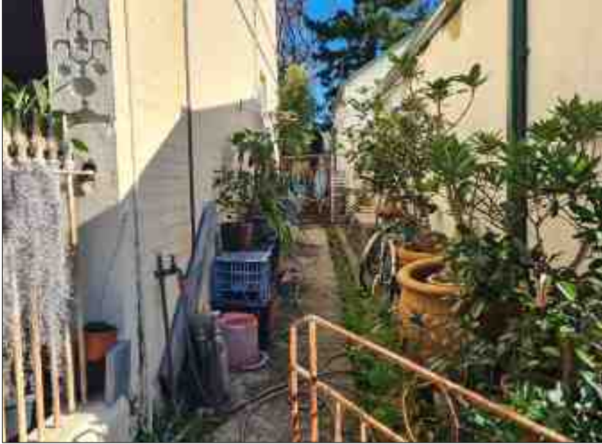
PHOTOGRAPH 13: RESIDENTIAL TERRACE (75 CROWN ST)
