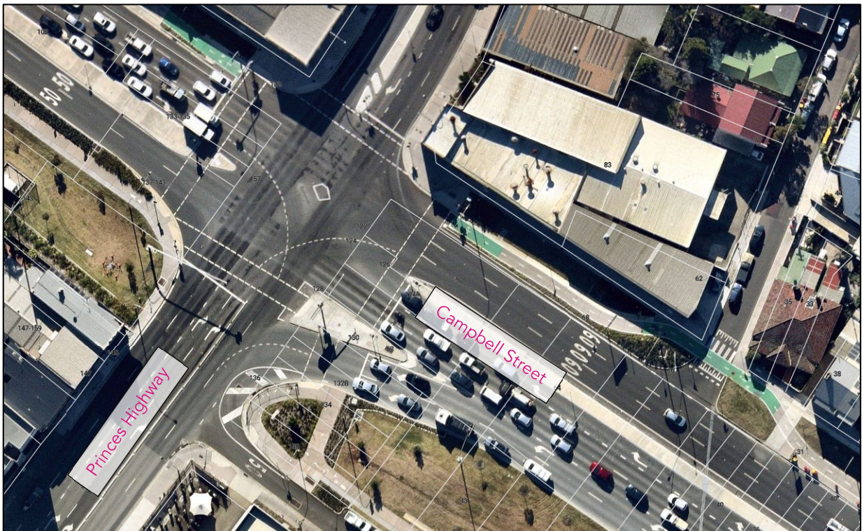
Figure 5 - Princes Highway / Campbell Street after upgrades (17 June 2021)
