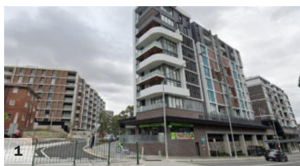
9-storey development on the Petersham RSL site
