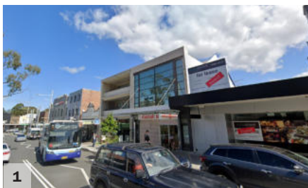
Southern Norton Street commercial properties
