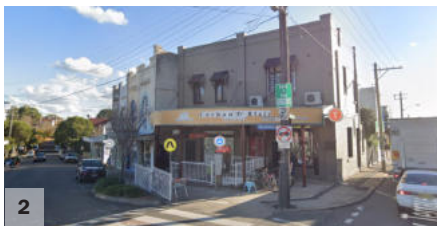
Commercial buildings on Victoria Street
