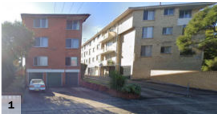
1 Existing walk-up flats at Loftus Street
