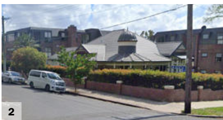
Development surrounding major heritage item on Julia Street
