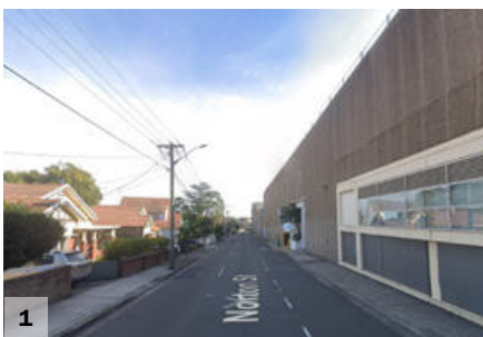
1 Norton Street interface with Ashfield Mall
