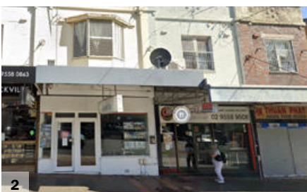
2 Illawarra Road (Google Maps)
