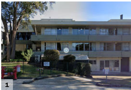
1 Presbyterian Aged Care facility on Charlotte Street
