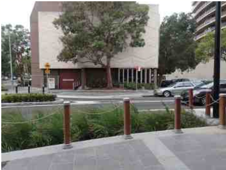
Figure 24 Chain and bollard fencing
