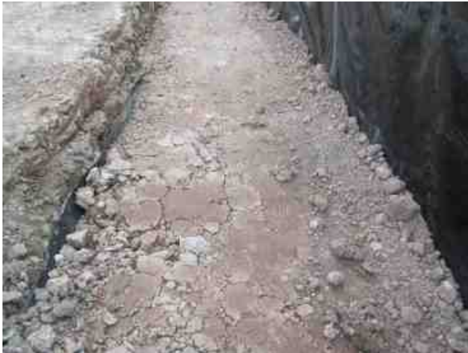
Figure 30 Compacted clay liner – note 1m depth of clay liner on trench face on left hand side of photo
