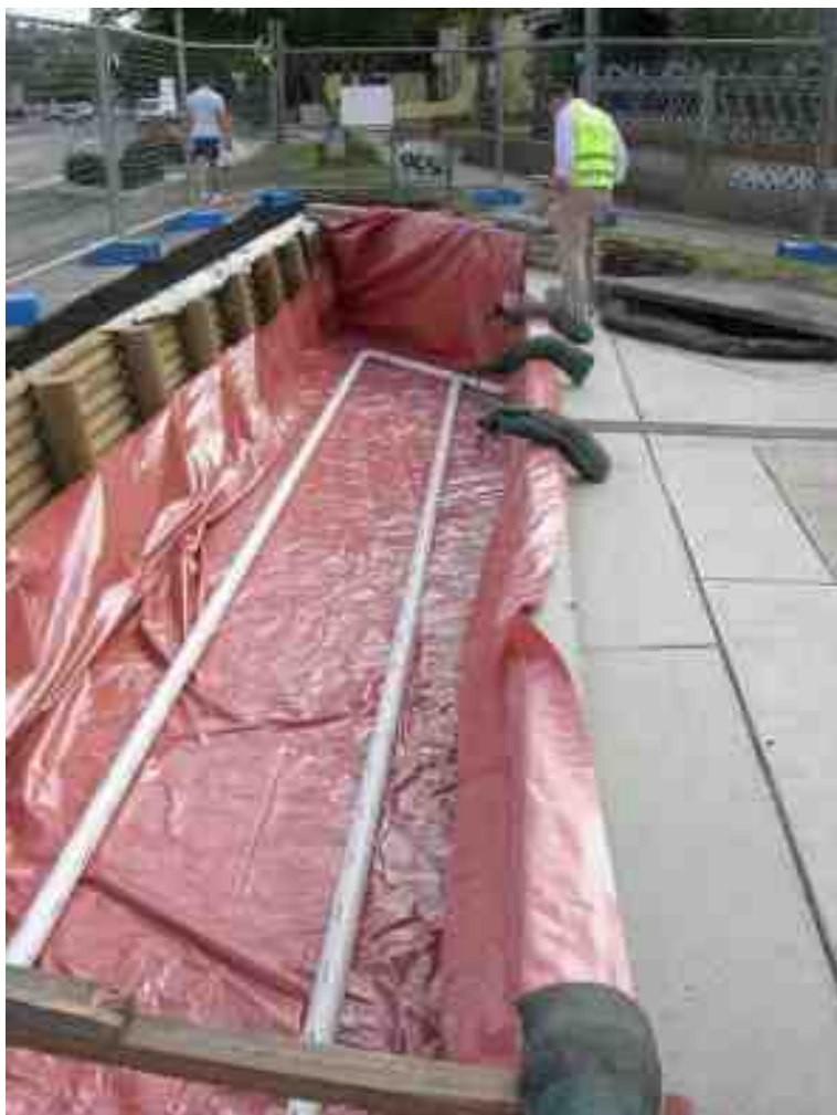
Figure 26 Bricks plastic liner and sub soil drains
