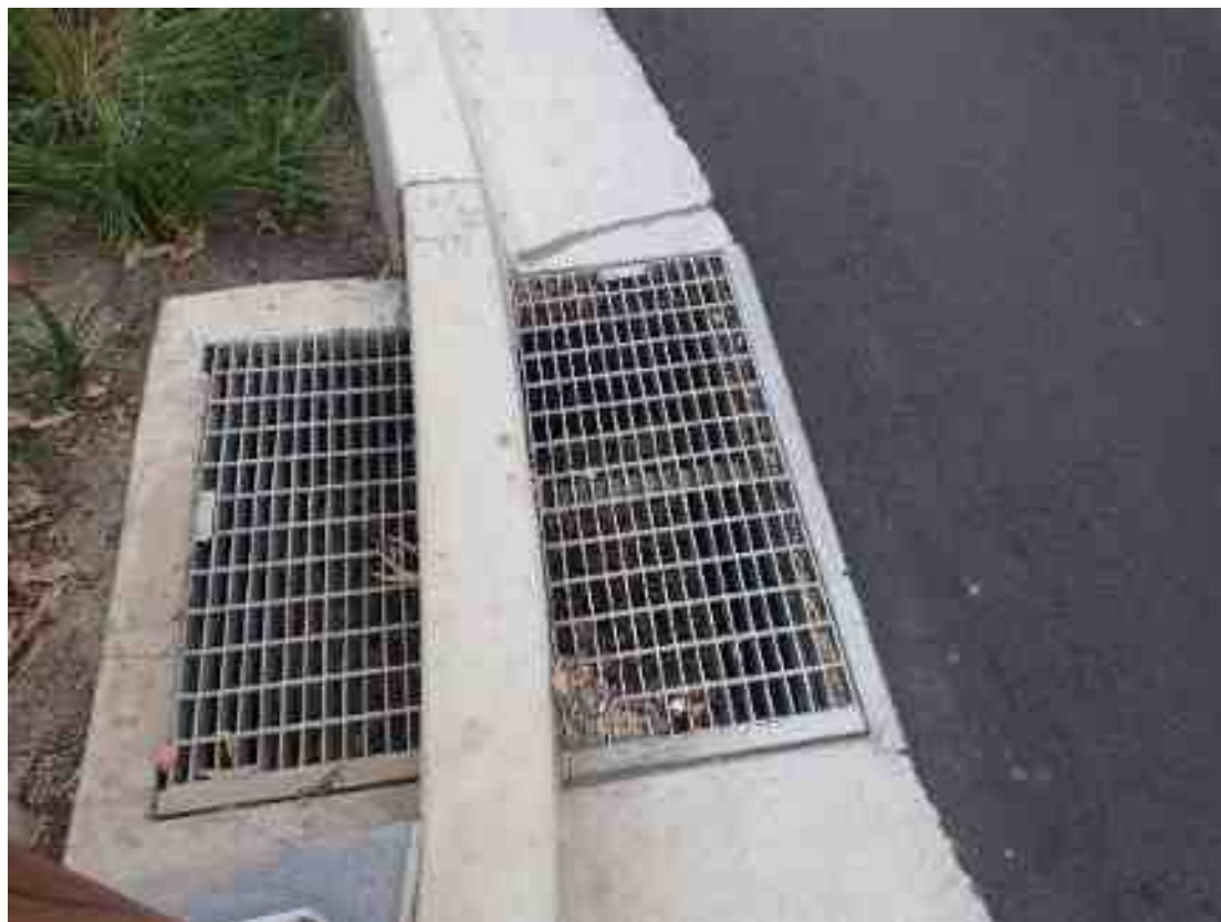
Figure 12 Double pit arrangements in streetscape rain garden
