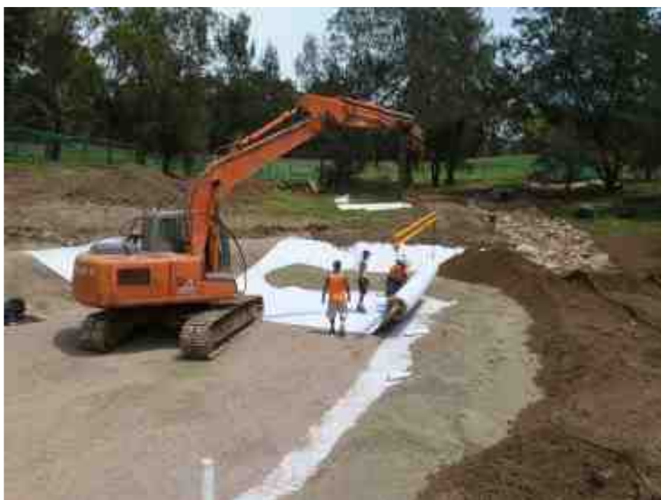
Figure 29 Geosynthetic clay liner being installed (note preparation of subgrade below liner which is free of any irregular rocks or sharp material)
