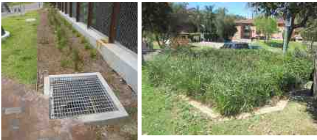
Figure 18 Steel edge (left) and concrete edge (right)
