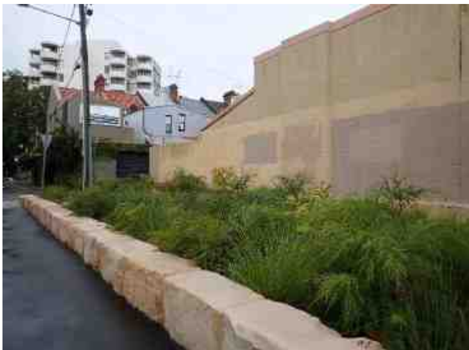
Figure 22 Sandstone wall which also functions as seating
