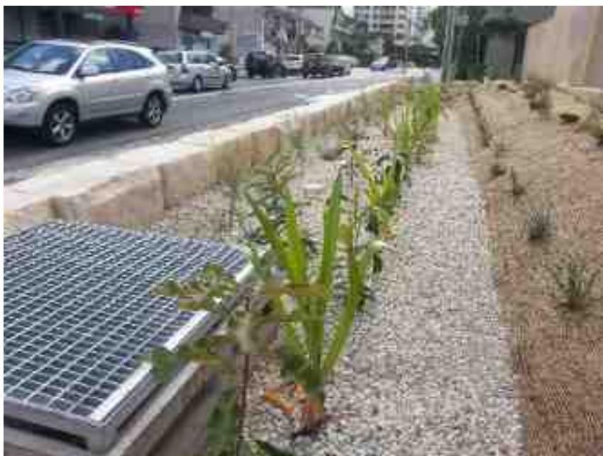
Figure 15 Clean no fines rock mulch to base of rain garden and jute mesh to batter slopes
