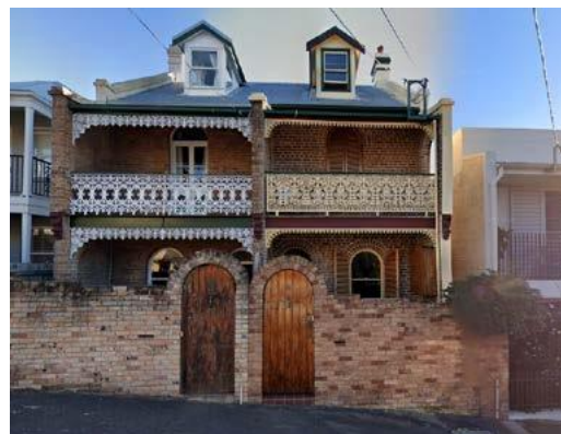
Example of two storey with attic window, Reuss St, Birchgrove
