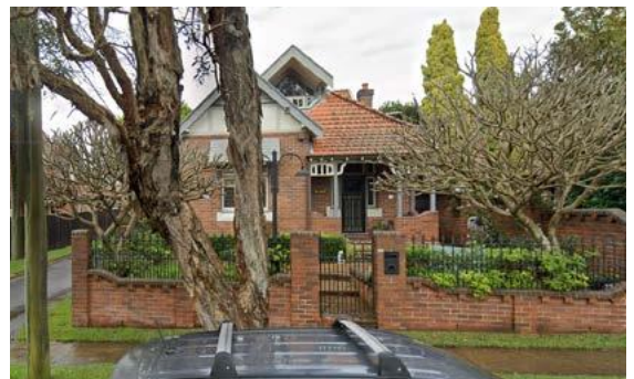
One storey frontage with second storey built into pitched roof with window facing street, Market St, Naremburn (7m HOB control)
