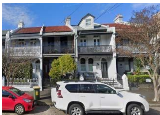
2-3 storey terraces, Darling St, Rozelle
