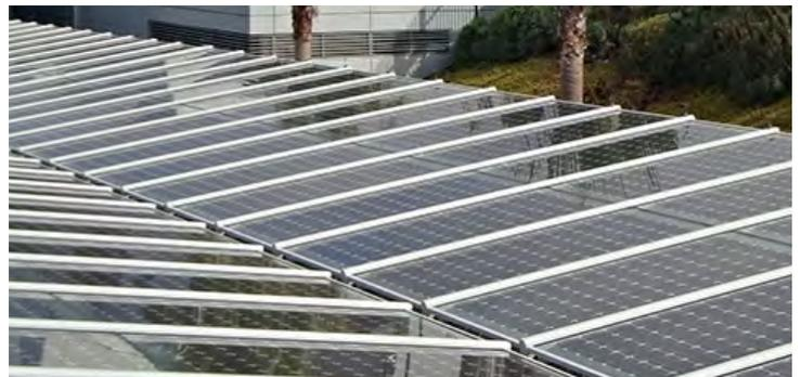
Photovoltaic solar shading structure to car park?<sup>7</sup>
