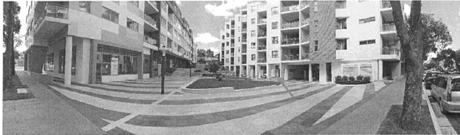
Image 4: Part of the mixed use development as viewed from Alice Street
