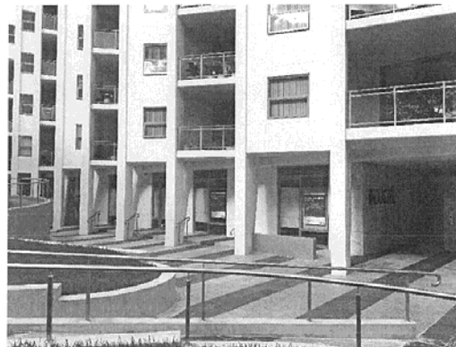
Image 5: Eastern façade of subject tenancies
