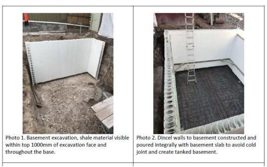
Photo 1 showing basement excavation during construction and foundation material.
