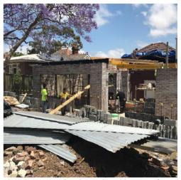
Photo 4. Structural timber and steel beams to first floor.
