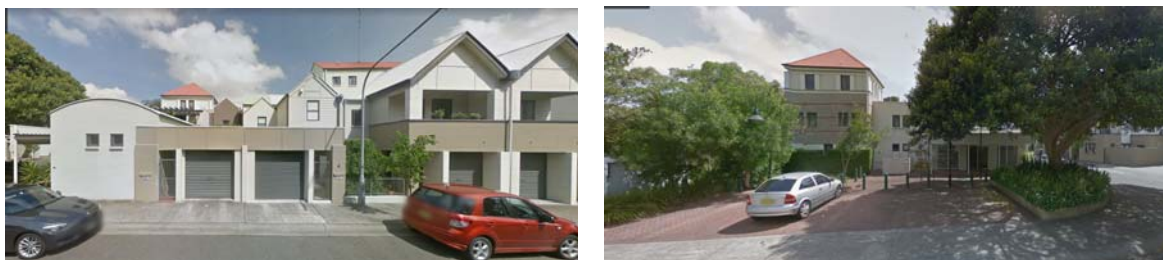
Figure 4: View of existing north-western (front) streetscape (left photo) and north-eastern streetscape (right photo) at McKell Street
