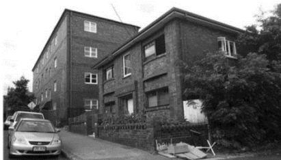
Figure 10: Residential flat buildings at and near the corner of Stanmore Rd and Tupper Street
