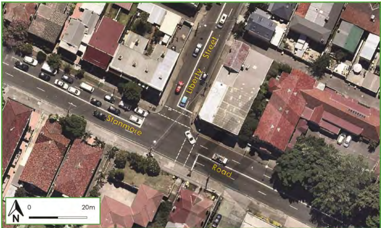
Figure 6: Aerial image of intersection of Stanmore Road and Liberty Street, Stanmore
