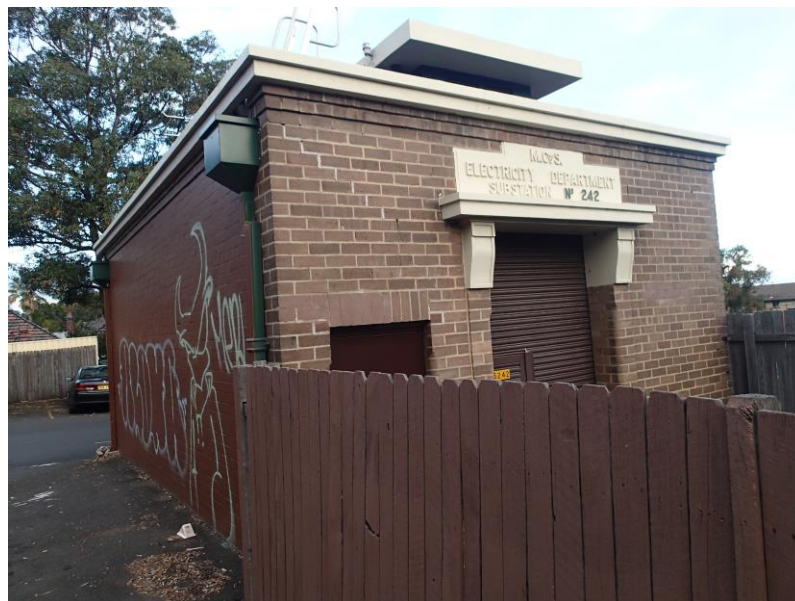
Figure 6: Electricity substation in Alma Avenue
