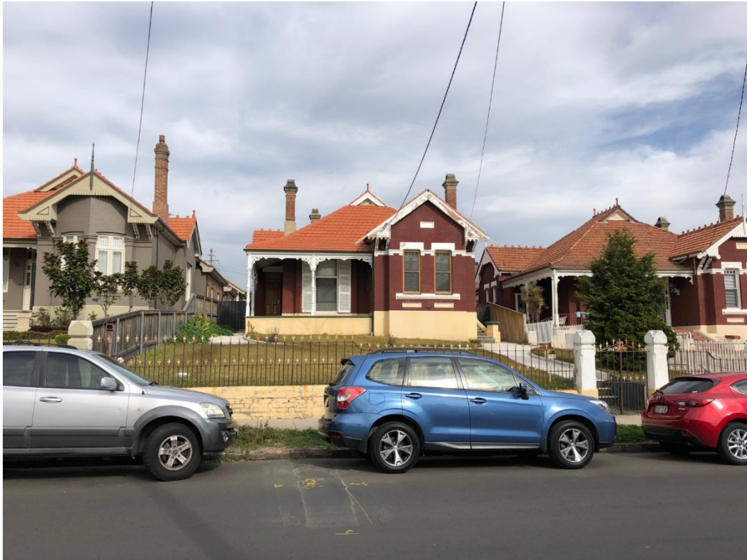
Picture 1 Site Photo – Smith Street frontage
