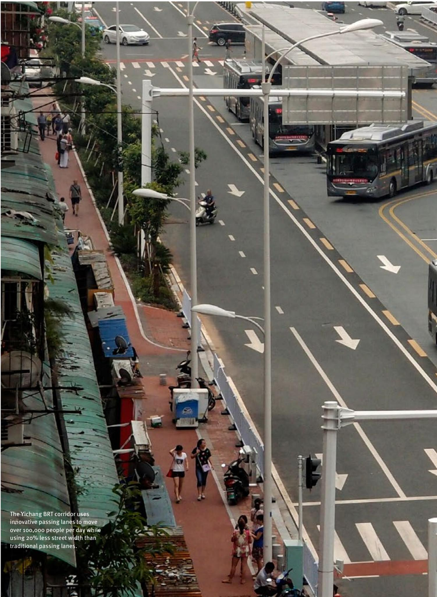
The Yichang BRT corridor uses innovative passing lanes to move over 100,000 people per day while using 20% less street width than traditional passing lanes.
