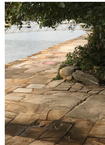
Relay the foreshore pathway to remove trip hazards and uneven surface
