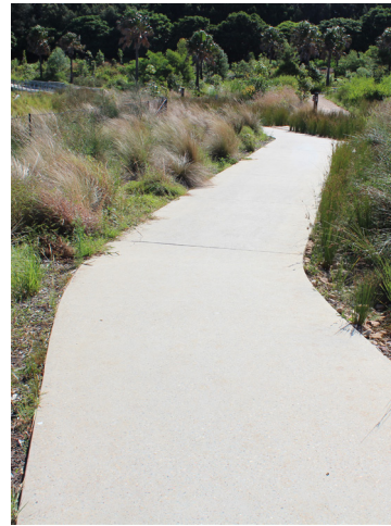
New 1.8m wide concrete pathway
