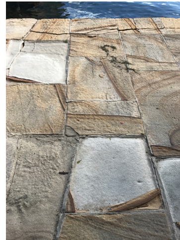
Relay the foreshore pathway to remove trip hazards and uneven surface
