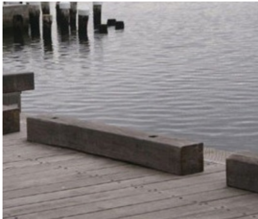
Large format timber sleepers as edge deterrents
