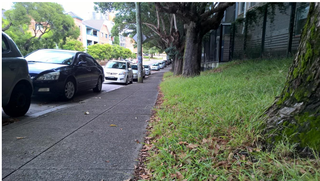
Photo 7: Trafalgar Street (west of Audley Street). Proposed widening of footpath (and associated kerb widening) to provide a 2.5m shared path by minor reduction in width of adjacent parking and traffic lanes.
