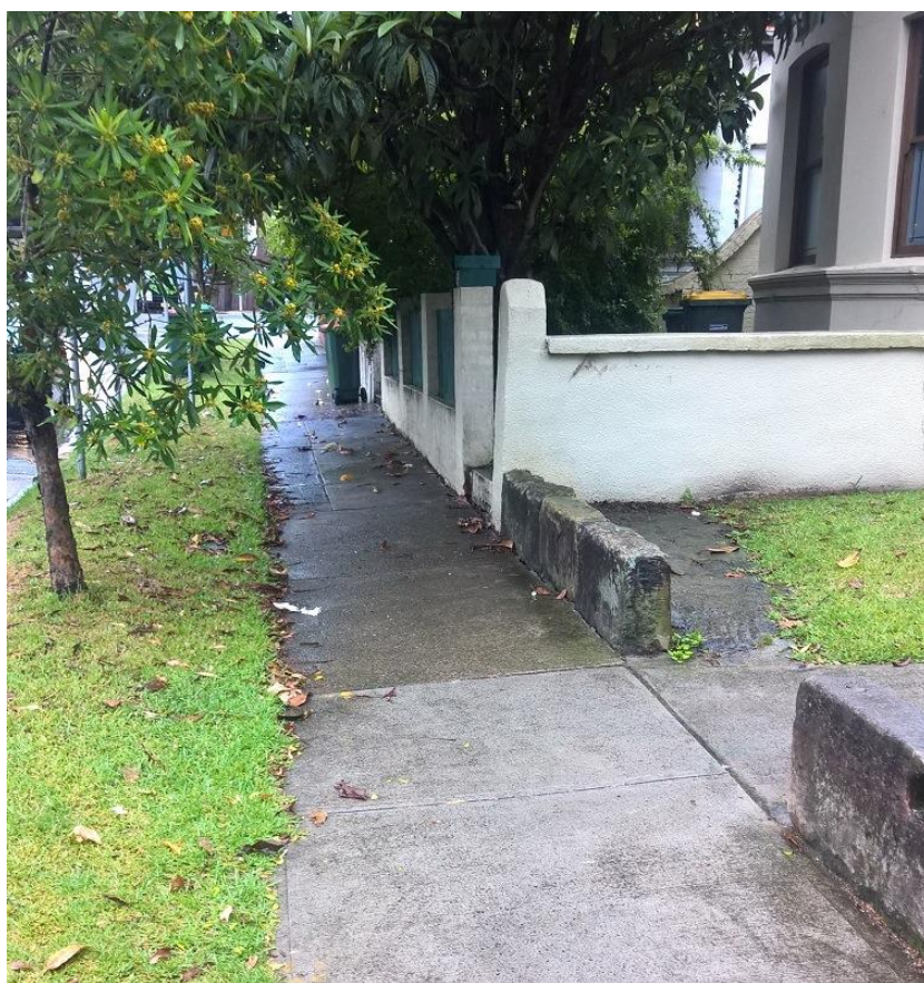
Photo 2: Old Canterbury Road (eastern side). Proposed widening of footpath to provide a 2.5m shared path (existing street trees to be replaced in remaining verge).
