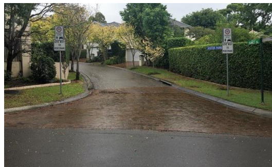
Figure 7.4: Entry Treatment – Textured Road Surface
