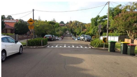
Figure 7.7: Road hump with planted kerb extensions
