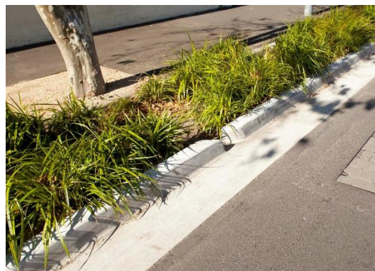
Figure 7.6: Rain Garden Kerb Extension
