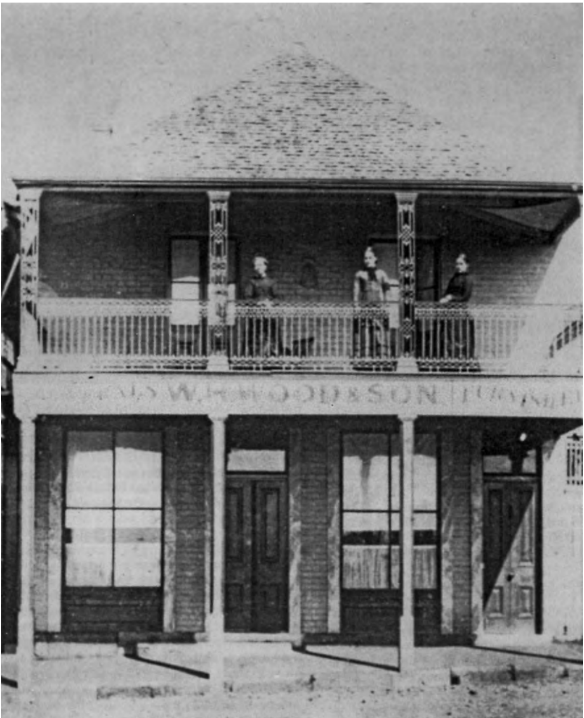
W H Wood & Son, 242 Darling Street, c1880s Built by William Henry Wood between 1860 and 1866, the shop/dwelling features a timber shingle roof, verandah with cast-iron grille columns and railings above a double-fronted shop front. The doorway at right gave access to the upper level. (Courtesy of J Greenwell)
