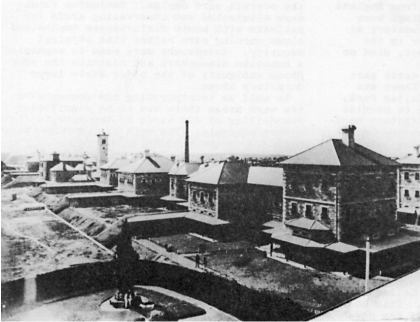
THE PAVILION WARDS, MALE DIVISION, AND WESTERN ELEVATION OF KIRKBRIDE BLOCK
