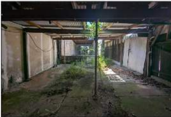
Easterly view of the open concreted and metal-roofed area. There is missing roofing and its northern wall is unfinished. The concrete is also in poor condition with considerable vegetation growing through its cracks.
