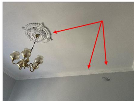
Figure 50. Modern ceiling roses and cornice in front bedroom. Distortion on the cornice can be seen from the former fireplace.
