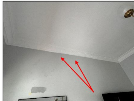
Figure 52. Red arrows indicating distortion on cornice as a result of eradication of former fireplace.
