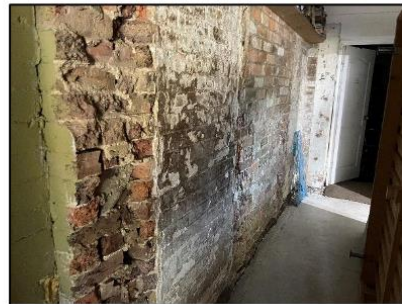
Figure 37. Internal view to the western wall, Lower Ground Floor. Note that some of these bricks are sandstock.
