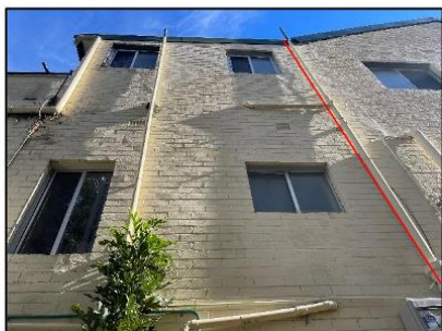
Figure 28. External view to the east elevation with the red line indicating the separation between the principal built form and the modified rear service wing. The modified rear service wing features stretcher bond masonry.
