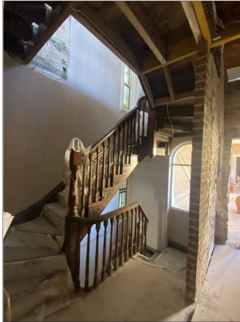
Figure 5.19 The stair and landing on the first floor. The stairwell retains two original leaded stair windows and an arched window added as part of the 1990s works. The opening to the rear wing also remains, however, a lightweight wall has been added to the former kitchen.
