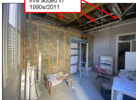
Figure 5.13 The lightweight framing added to the central wall.
