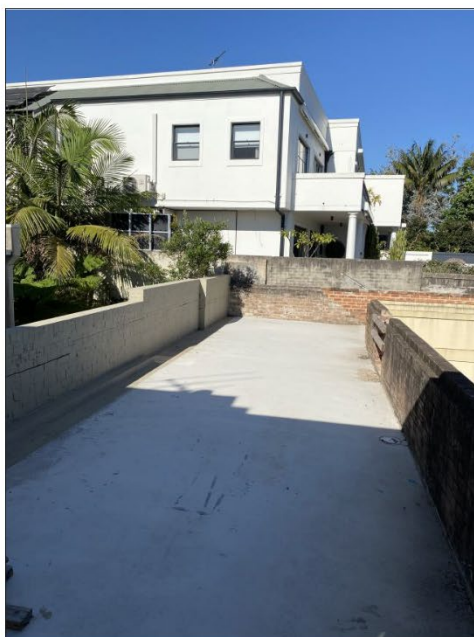
Figure 5.37 The new roof terrace and slab (part of the 2019 approval) which replaced the 1990s pitched roof.
