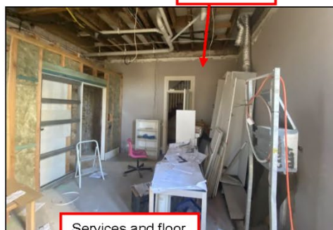
Figure 5.12 The second, main ground floor room. The door from the hall and toplight remains, however, the modern floor and ceiling linings have been removed and reveal a concrete floor slab and sheeted flooring and kitchen services previously added over the space.
