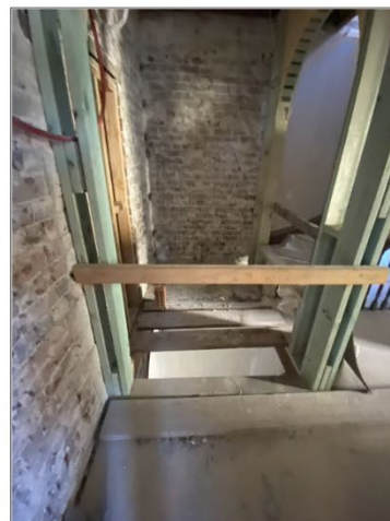
Figure 5.20 The two roomed layout and early brick cross wall remains, however, some flooring has been removed to create a void over the ground floor hall.
