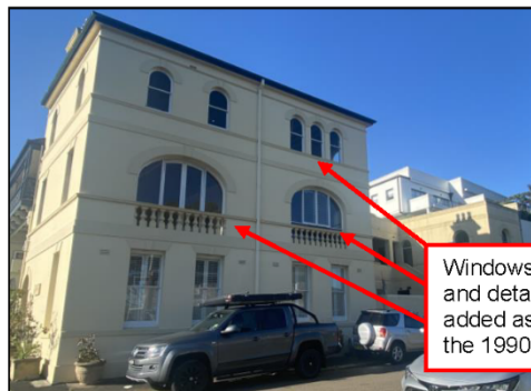
Figure 5.4 The Bates Street façade of the main wing. The large arched openings on the first floor were infilled and windows were reinstated to the second floor as part of the 1990s works.
