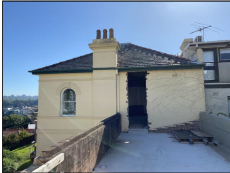
Figure 5.38 The upper, western façade of the main wing. The new slab has an opening for the approved lift.
