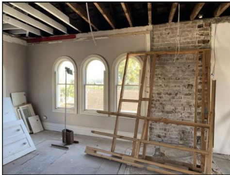
Figure 5.35 The trio of windows on the Bates Street façade. The two eastern windows were reinstated as part of the 1990s works. The floor retains evidence of various changes, patching and repairs and addition of services.
