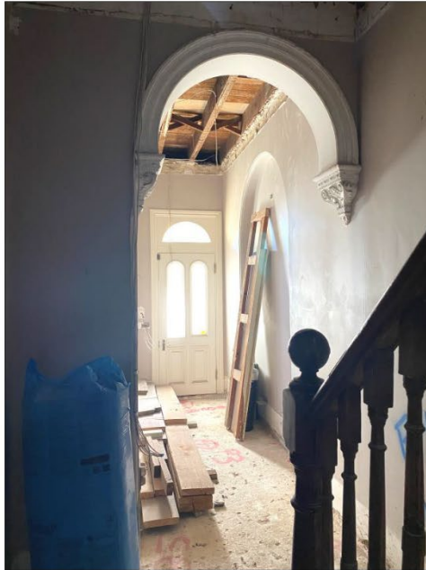
Figure 5.8 The building entry and side hall which retains a blind, recessed arch in the southern party wall, hall arch and door openings with toplights.
