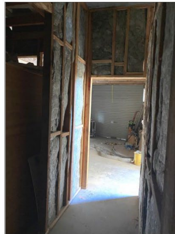
Figure 5.18 The existing garage which was added as part of the 1990s works. Some lightweight framing has been recently added.
