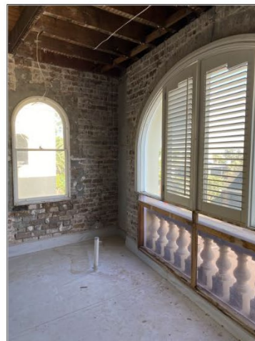
Figure 5.26 The modern kitchen fitout and ceiling have been removed from the second room, however, the windows and details added as part of the 1990s works remain. The floor has modern sheeting. Some lightweight walls have been recently added.
