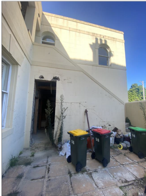
Figure 5.7 The western arm of the rear wing including the external stair were added as part of the 1990s works. A new opening has been recently made at ground floor level.
