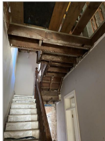
Figure 5.16 The linings and part of the ceiling over the hall have been removed. An opening adjacent to the stair accesses the rear wing.
