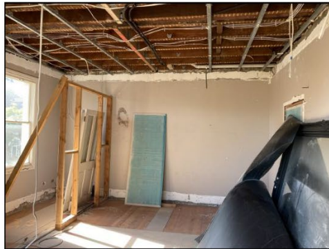
Figure 5.21 The front (eastern) room on the first floor (former living room). The modern ceilings, cornices and joinery have been removed, however, the fireplace, timber floors, windows and doors remain.
