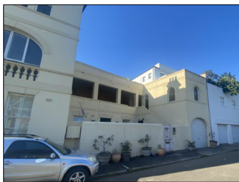
Figure 5.5 The early two storey rear wing was extended and modified as part of the 1990s works. The works included the addition the garage constructed to the Bates Street frontage with bedroom and services areas over connected by the open, but covered terrace. An external stair also extends up from the courtyard to the first floor. The high boundary (courtyard) wall was also modified as part of the 1990s works.
