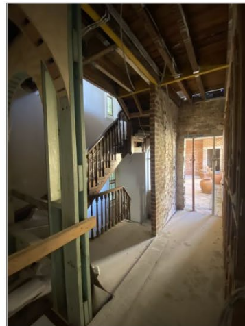
Figure 5.20 The two roomed layout and early brick cross wall remains, however, some flooring has been removed to create a void over the ground floor hall.
