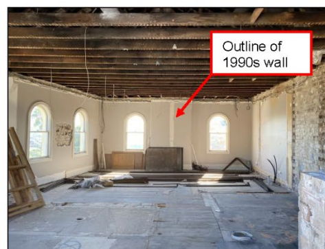
Figure 5.30 The second floor of the main wing has been recently opened up and modern linings and details removed. The outline of the wall relocated as part of the 1990s works (below) remains on the breast on the eastern wall. No fireplace was existing. The early cross wall also the robes, ensuite and associated finishes added as part of the 2011 works have also been removed. The patched, repaired and modified floor indicates the various changes.
