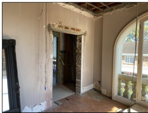
Figure 5.25 An existing door in the cross wall between the two rooms has been widened.
