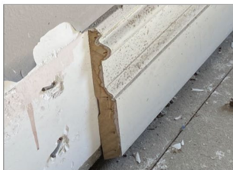
Figure 5.34 The skirtings and timber joinery are modern and have been previously replaced.
