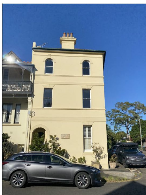
Figure 5.2 The eastern, Ballast Point Road façade. The front wing is constructed to both street frontages. The primary facades retain rendered wall finish and decorative mouldings, square and arched headed openings and timber framed windows and doors.
