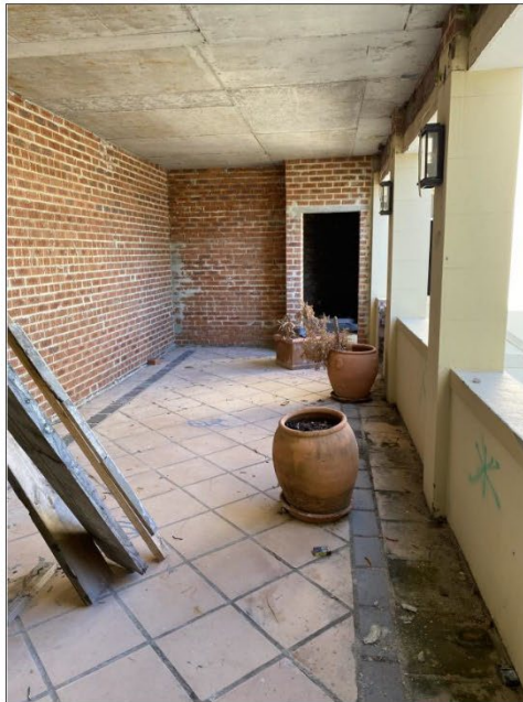
Figure 5.27 The first floor terrace in the rear wing. An opening has been made in the existing floor slab to accommodate the lift and new brick walls and a concrete slab have been added (as approved, 2019).
