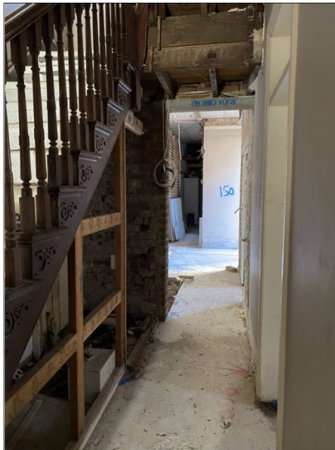
Figure 5.16 The linings and part of the ceiling over the hall have been removed. An opening adjacent to the stair accesses the rear wing.
