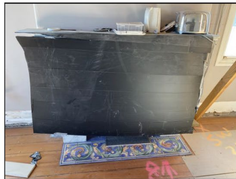
Figure 5.23 The floor patching and modified fireplace hearth undertaken as part of the 1990s works is evident. The fireplace also remains and has been covered.
