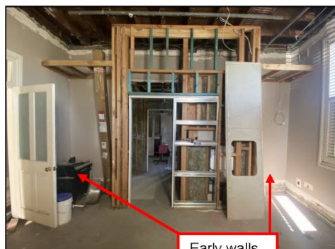
Figure 5.11 The two roomed layout and wall between the two main ground floor rooms remain. However, lightweight framing has been added in the existing wide opening.
