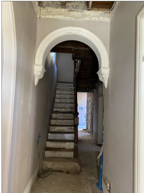
Figure 5.15 The side hall retains the original timber stair and timber balustrade and details which were repaired as part of the 1990s works.
