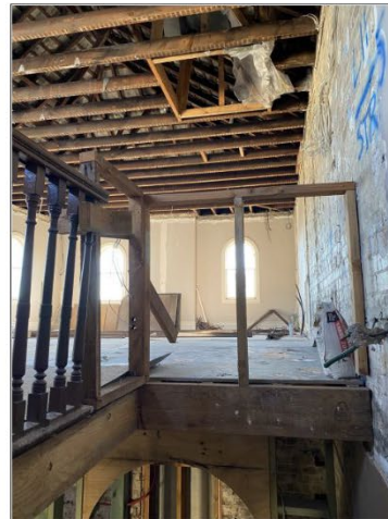
Figure 5.30 The second floor of the main wing has been recently opened up and modern linings and details removed. The outline of the wall relocated as part of the 1990s works (below) remains on the breast on the eastern wall. No fireplace was existing. The early cross wall also the robes, ensuite and associated finishes added as part of the 2011 works have also been removed. The patched, repaired and modified floor indicates the various changes.
