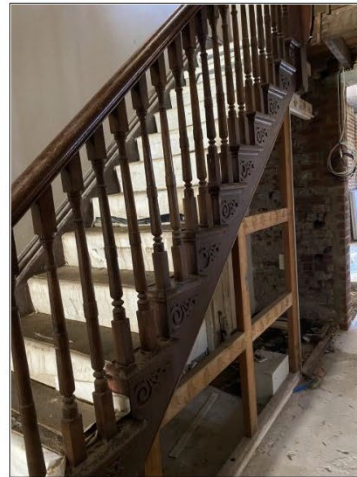
Figure 5.16 The linings and part of the ceiling over the hall have been removed. An opening adjacent to the stair accesses the rear wing.
