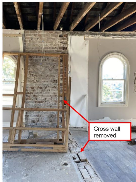
Figure 5.30 The second floor of the main wing has been recently opened up and modern linings and details removed. The outline of the wall relocated as part of the 1990s works (below) remains on the breast on the eastern wall. No fireplace was existing. The early cross wall also the robes, ensuite and associated finishes added as part of the 2011 works have also been removed. The patched, repaired and modified floor indicates the various changes.
