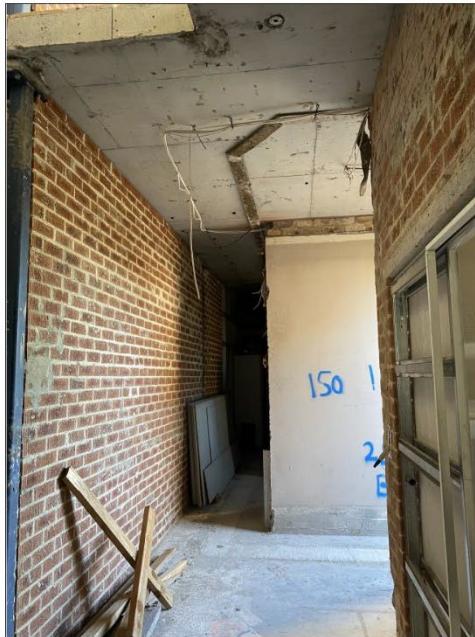
Figure 5.17 The rear wing which was extended and altered as part of the 1990s works. Openings have recently been made in the slabs to accommodate the approved lift. Some alterations to the existing bathroom and study have also been undertaken.
