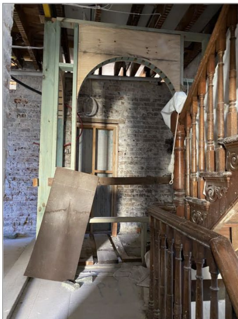
Figure 5.20 The two roomed layout and early brick cross wall remains, however, some flooring has been removed to create a void over the ground floor hall.
