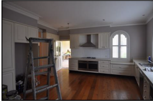
Figure 3.30 The renovated kitchen area on the first floor. The removal of the internal walls and balcony appears to have resulted in the addition of a new ceiling and some patching of the floor. An opening was also made to access the terrace over the rear wing.
