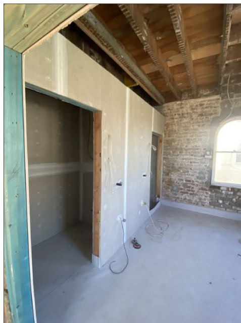
Figure 5.26 The modern kitchen fitout and ceiling have been removed from the second room, however, the windows and details added as part of the 1990s works remain. The floor has modern sheeting. Some lightweight walls have been recently added.
