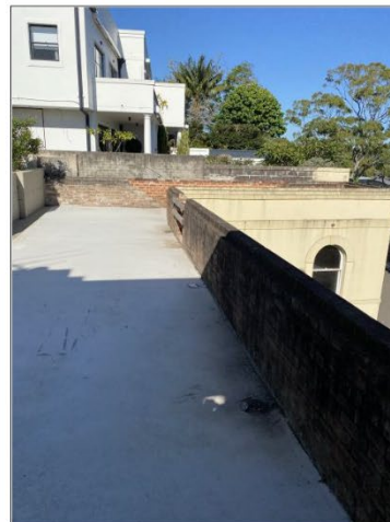
Figure 5.37 The new roof terrace and slab (part of the 2019 approval) which replaced the 1990s pitched roof.
