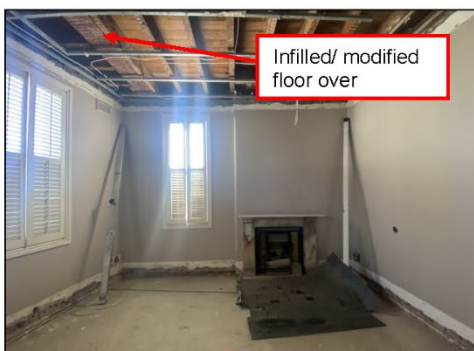
Figure 5.10 The front, ground floor retains the window openings and windows. Evidence of the first floor infill/ patching is visible over the northern side.
