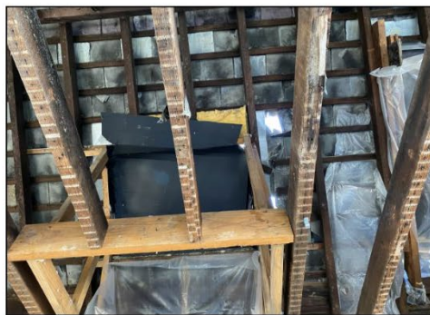
Figure 5.32 Roof framing and cladding and existing skylight framing.
