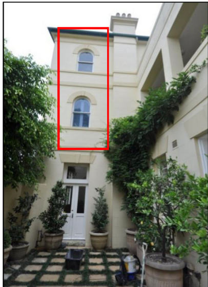
Figure 3.26 The walls facing the courtyard c. 2016 showing the windows, rendered finish and details added as part of the 1990s works.
