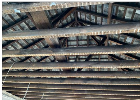
Figure 5.33 The roof framing and slate cladding. Some repairs are evident.
