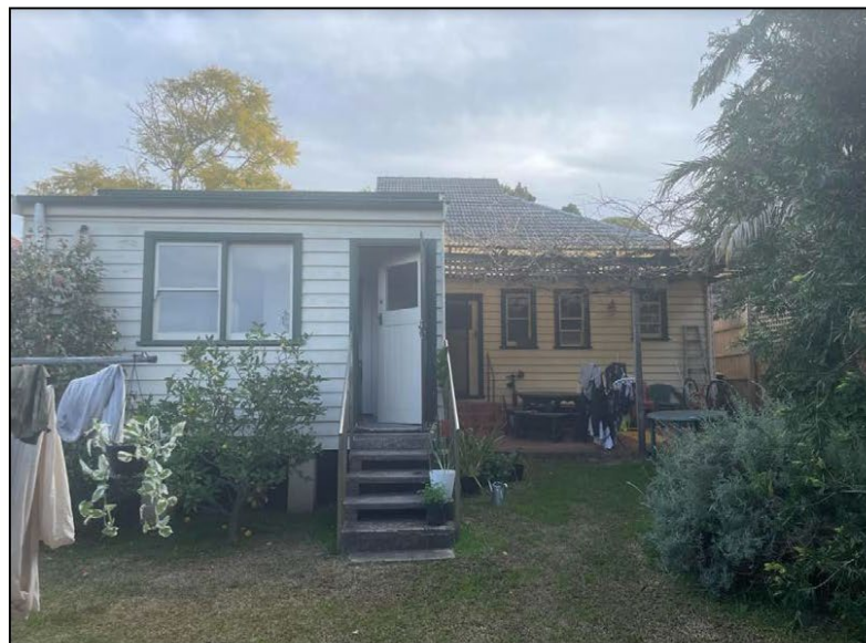
Figure 9: View of rear weatherboard extension.
