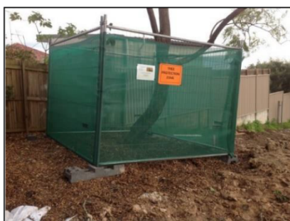
Figure 4: Tree Protection Fencing
