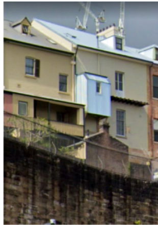
Two "pod additions" to State Heritage listed terrace houses at Lower Fort Street visible for Pottinger Street and Parbury Lane to solve the same issue of adding needed bathrooms to items of heritage.
