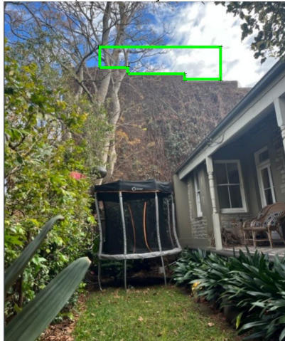
Figure 4: existing featureless wall of the structure at No. 215 Lilyfield Road, as viewed from the adjoining property to the east, No. 213 Lilyfield Road. Source: No. 213 Lilyfield Road neighbour submission.
