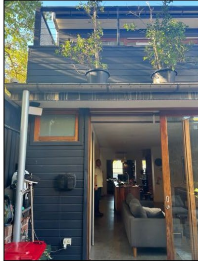
Figure 14: Left hand side of rear elevation.
