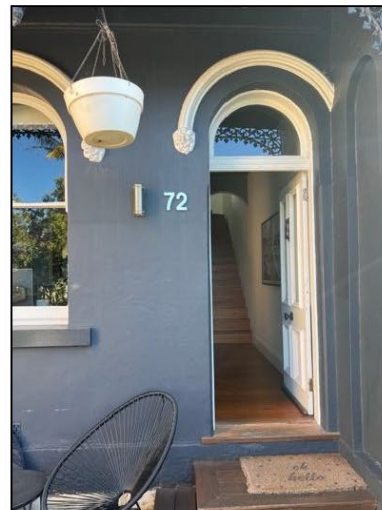
Figure 13: Partial view of principal elevation.
