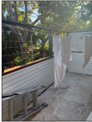
Figure 29: Existing rear balcony.
