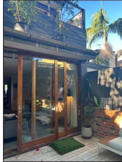
Figure 15: Right hand side of rear elevation.
