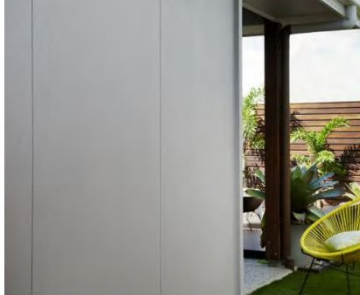
Roof terrace Cladding – Fibre Cement (FC2)– Easylap Panel – Dulux ivory
