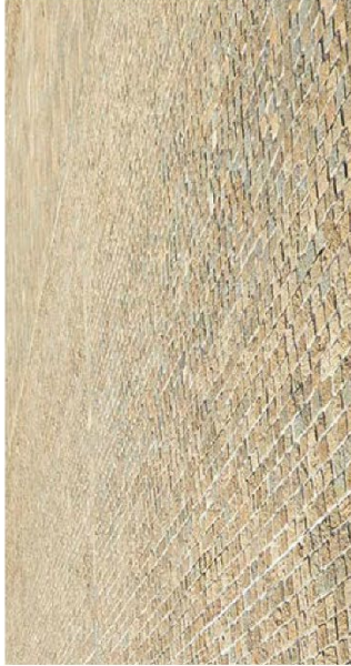
UNIT PAVING MATERIAL: GRANITE - BLUESTONE PAVERS WHARF ROAD AND MILITARY DRIVE SHARED ZONE
