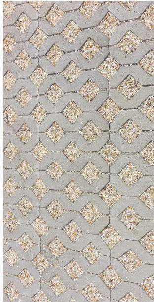
PERMEABLE GRID PAVERS MATERIAL: PRECAST CONCRETE WITH GRAVEL INFILL CAR PARK SPACES
