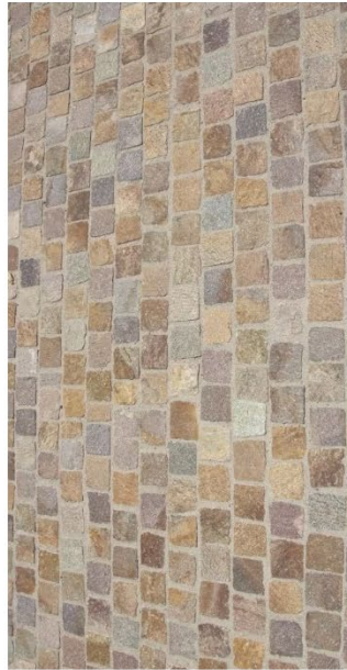
UNIT PAVING MATERIAL: GRANITE - TORONTO PAVERS WHARF ROAD AND MILITARY DRIVE SHARED ZONE
